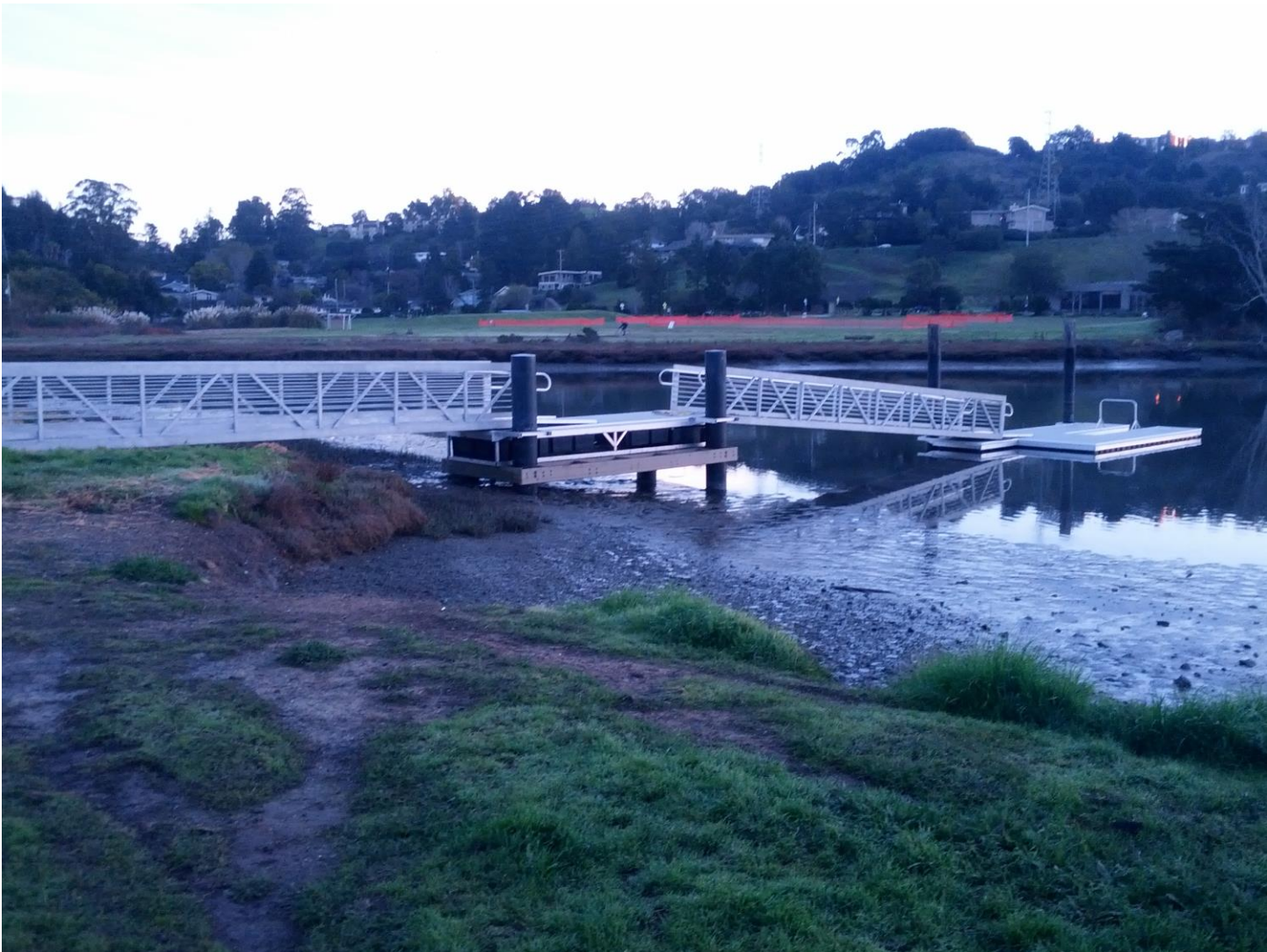
Figure 2: Photograph of New Dock (AFTER PROJECT)
