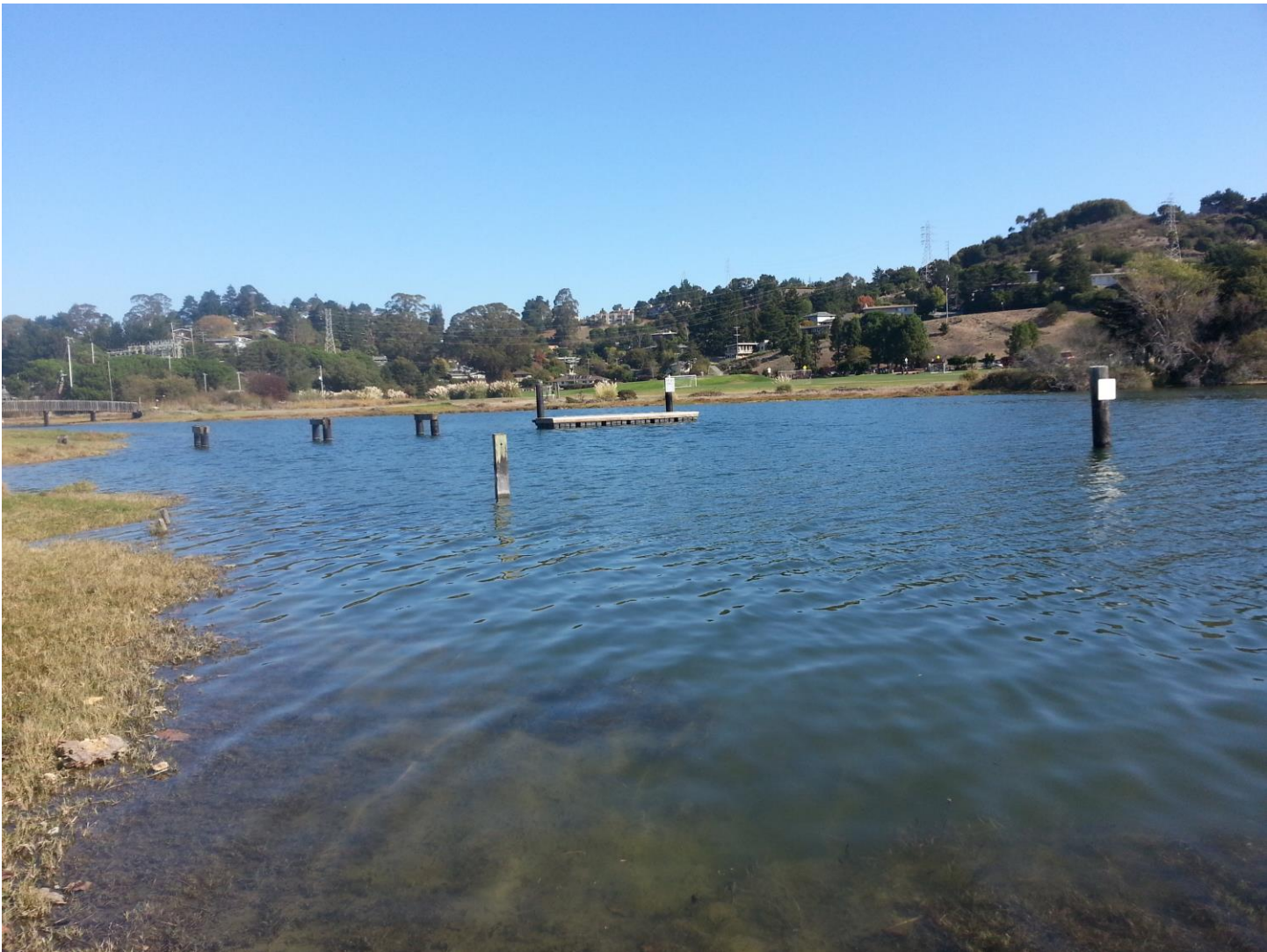
Figure 1: Photograph of Old Dock (BEFORE PROJECT)
