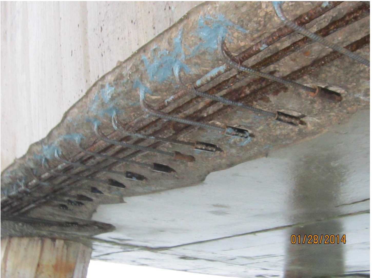
Figure 3: After chipping-away the loose concrete, the most seriously damaged reinforcing was replaced. These angled pieces of rebar were epoxied into holes drilled up into the outer wall of the beam, and they are coupled to existing bars that had been cut back to competent steel. (Photo by Ramon Bernardo)
