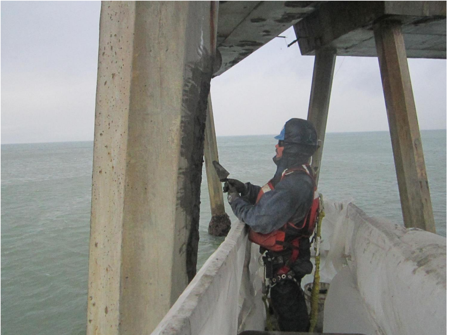
Figure 6: The spalled concrete on the piles was replaced with waterproof mortar.
