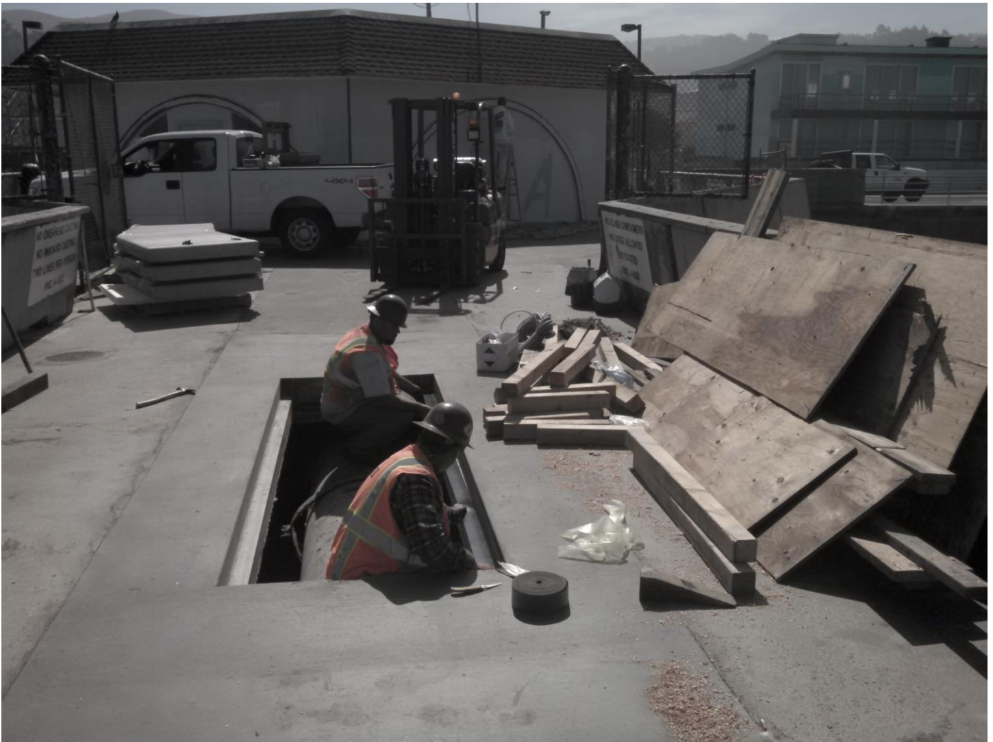
Figure 7: The crew is just completing the replacement of a portion of deck that would support the new pre-cast concrete hatch units, which are stacked on dollies at the left rear of the photo. (Photo by Lee Panza)
