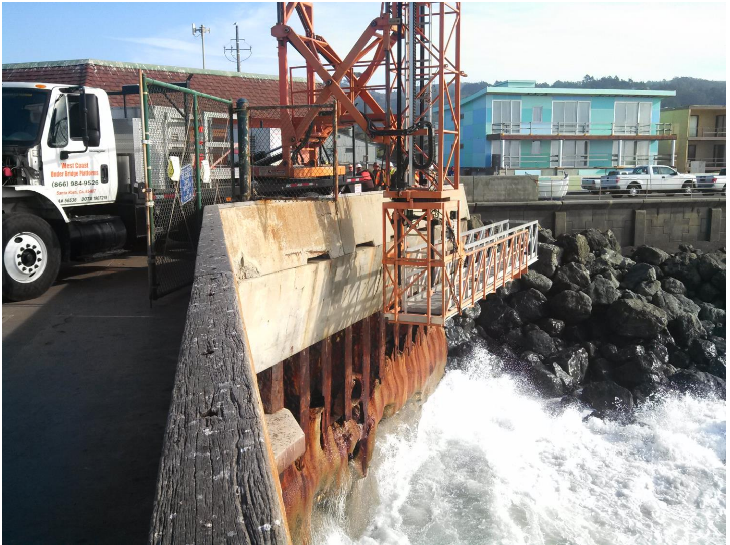
Figure 1: Upon delivery of the scaffold truck, and before it was driven out onto the Pier to begin the work, the scaffolding was checked-out. This machine allowed the crew to work safely on the underside of the Pier (the platform section can swing around to any angle underneath) and on the piles. A boat or barge could not have worked between the piles and in the surf zone. (Photo by Lee Panza)
