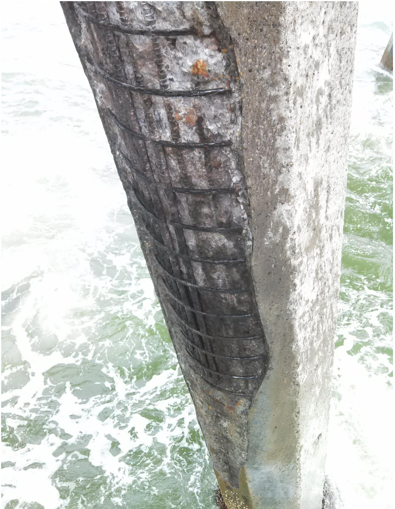
Figure 5: On the deteriorating piles, the loose concrete was chipped away, but the reinforcing was found to be still in reasonable condition; it was wire-brushed clear of rust. (Photo by Lee Panza)
