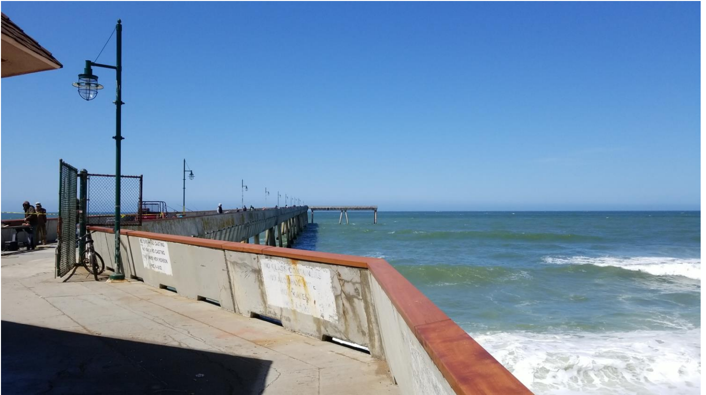
Figure 9: New lumber, of a type that is so tough and durable it is used for truck beds, was fitted and bolted down to the walls. The lighting fixtures were all replaced with LED units. (Photo by Lee Panza)
