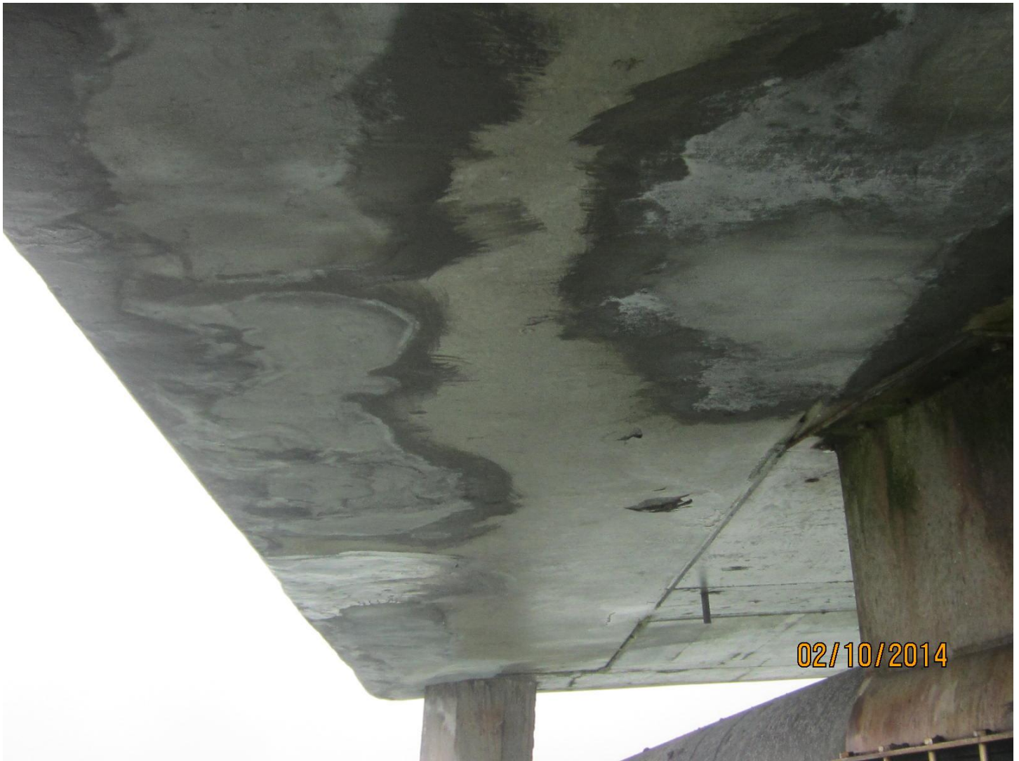
Figure 4: After replacing the damaged steel reinforcement, the spalled areas were filled and sealed with waterproof mortar. (Photo by Ramon Bernardo)
