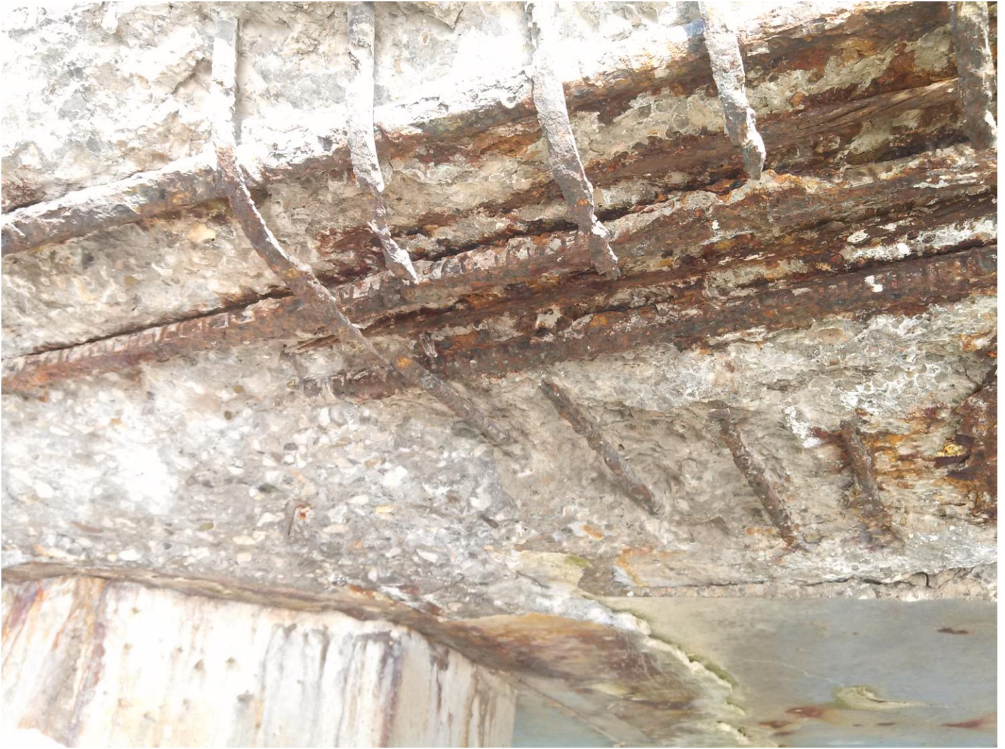
Figure 2: Spalling of the concrete had exposed the reinforcing, and many of the outer bars had rusted completely through. (Photo by Lee Panza)
