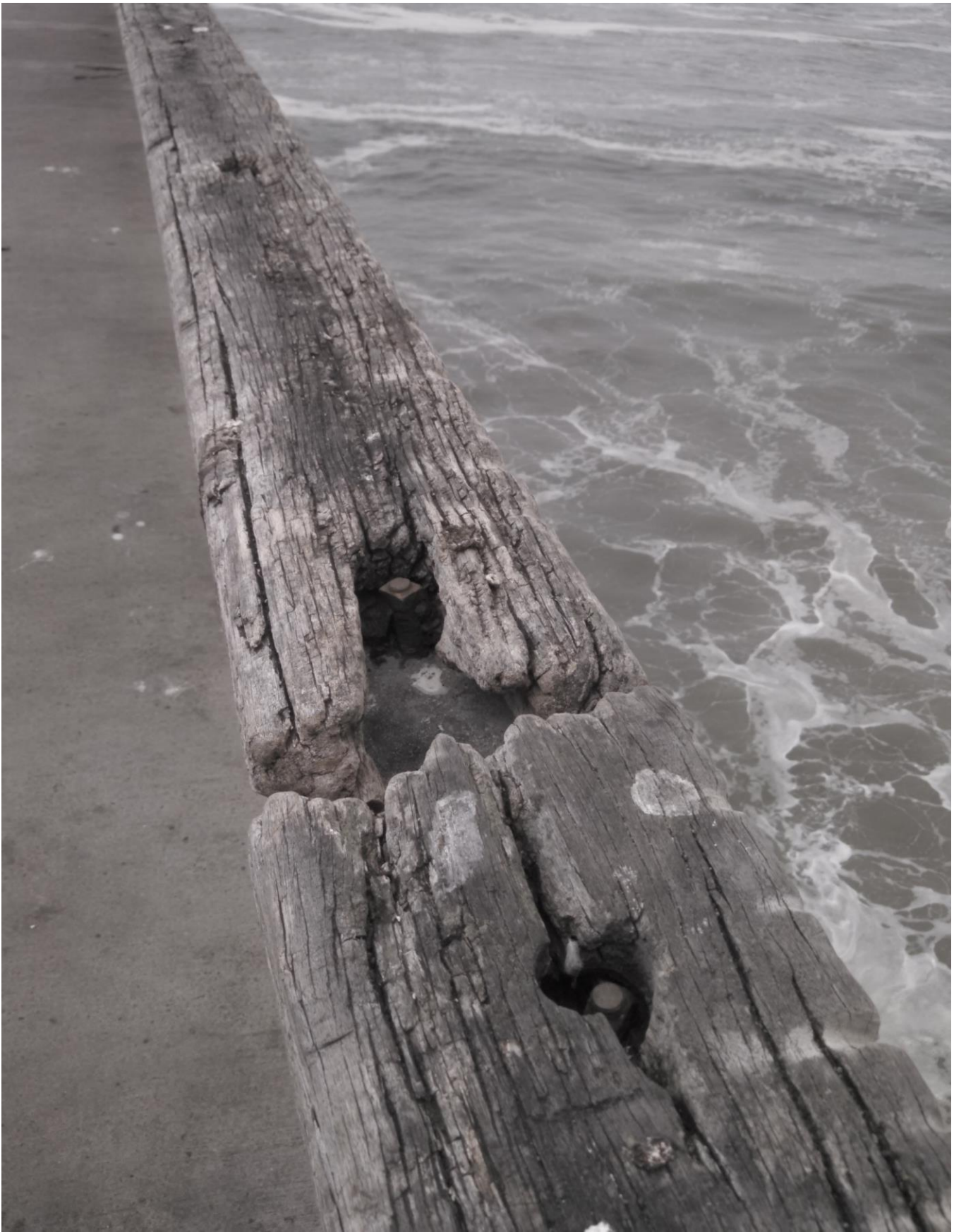
Figure 8: The wood caps on the parapet wall guardrails had deteriorated to such an extent that some had already fallen off and those remaining were not much better off. (Photo by Lee Panza)
