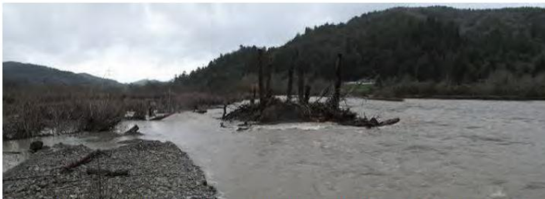
Figure 2. Looking downstream at Terwer ELJ 1 and willow baffles protecting a side channel and Holocene soils and creating low velocity habitat (01/01/10 - near bankfull event ~1,600 cfs).
