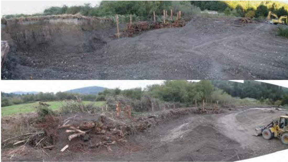
Figure 3. Looking downstream at an engineered log jam (Terwer Crib Wall Jam) in Terwer Creek during construction (Fall 2009).
