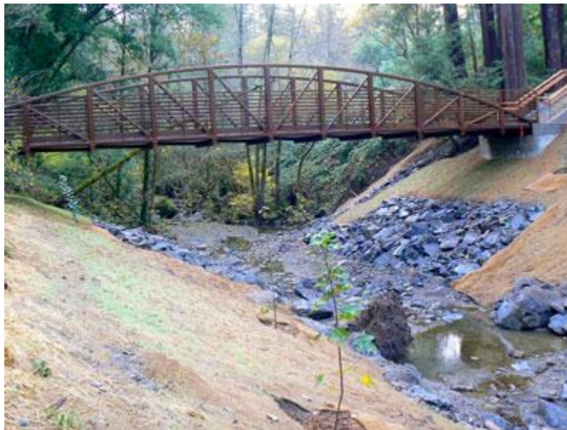
Dutch Bill Creek Fish Passage Improvement Project Photo: Gold Ridge Resource Conservation District
