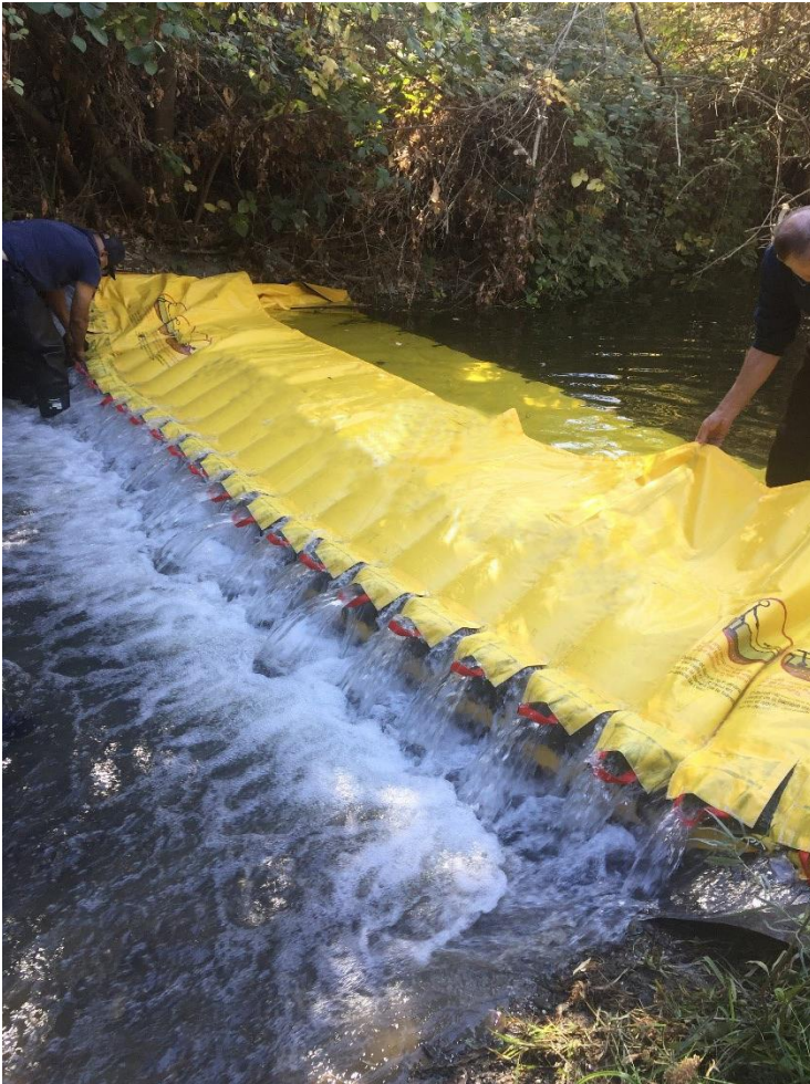
Figure 1-4: Commercial Underflow Dam
