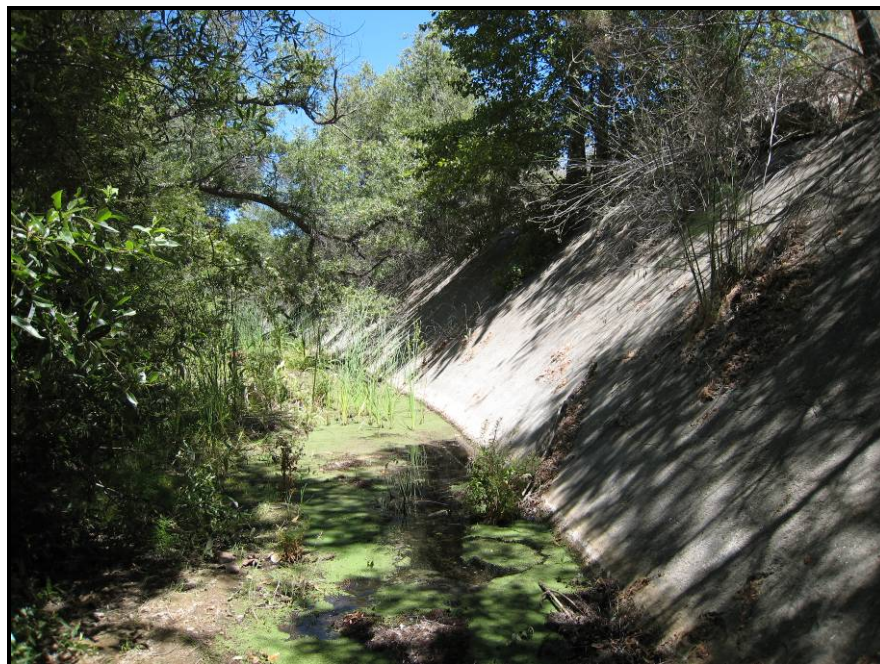
Figure 3 – Looking upstream from the crossing. Note concrete revetment wall on right bank. The left bank is natural and vegetated with dense riparian plants.
