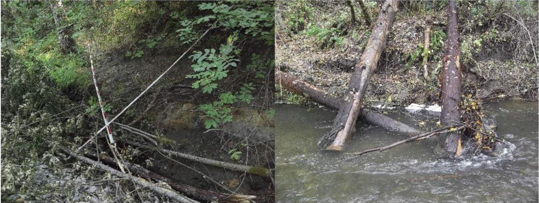
Site 1 before (left) and after (right) treatment. Stadia rods in pre-treatment photo indicate log placement within the site. Photos were taken from the left bank facing across the channel.
