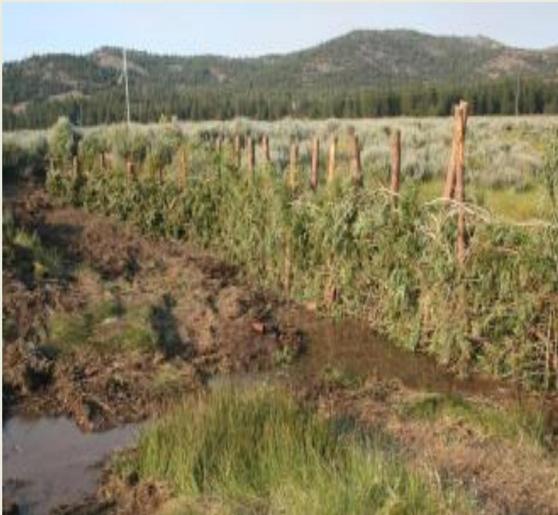
Restoring Hydrologic Function: TSF has installed four BDAs at select instream locations between engineered check dam structures on two sub-channels. Additional BDAs will be installed on Dixie Creek in 2019. The combination of these structures will slow the flow of water through the meadow and reconnect the stream to the floodplain, resulting in increased sediment and nutrient deposition, as well as improved habitat for native plant and animal species.
