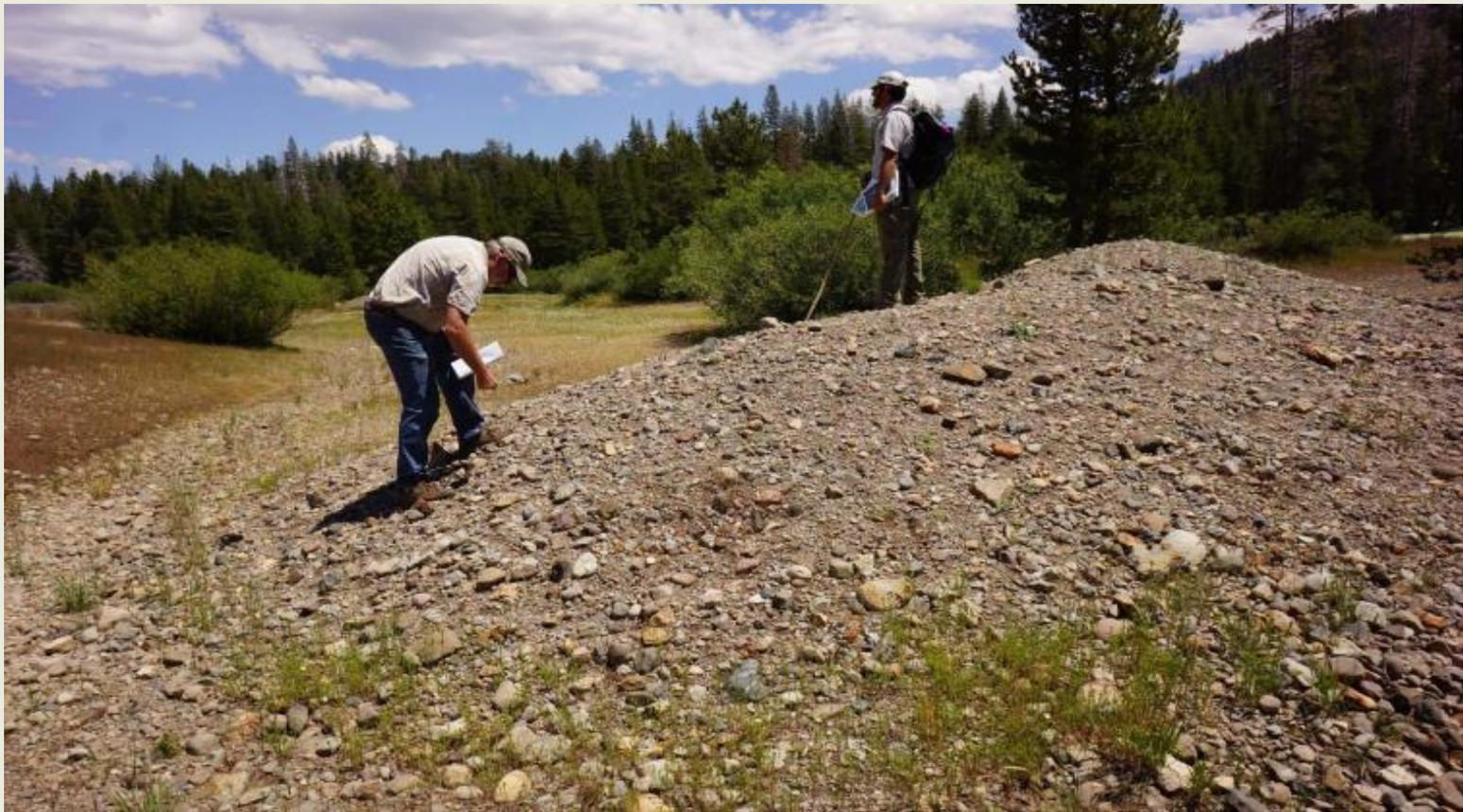
Gravel push-up dam in the historic channel of Lacey Creek through Upper Lacey Meadow, used to divert the stream into the present day unstable channel.
