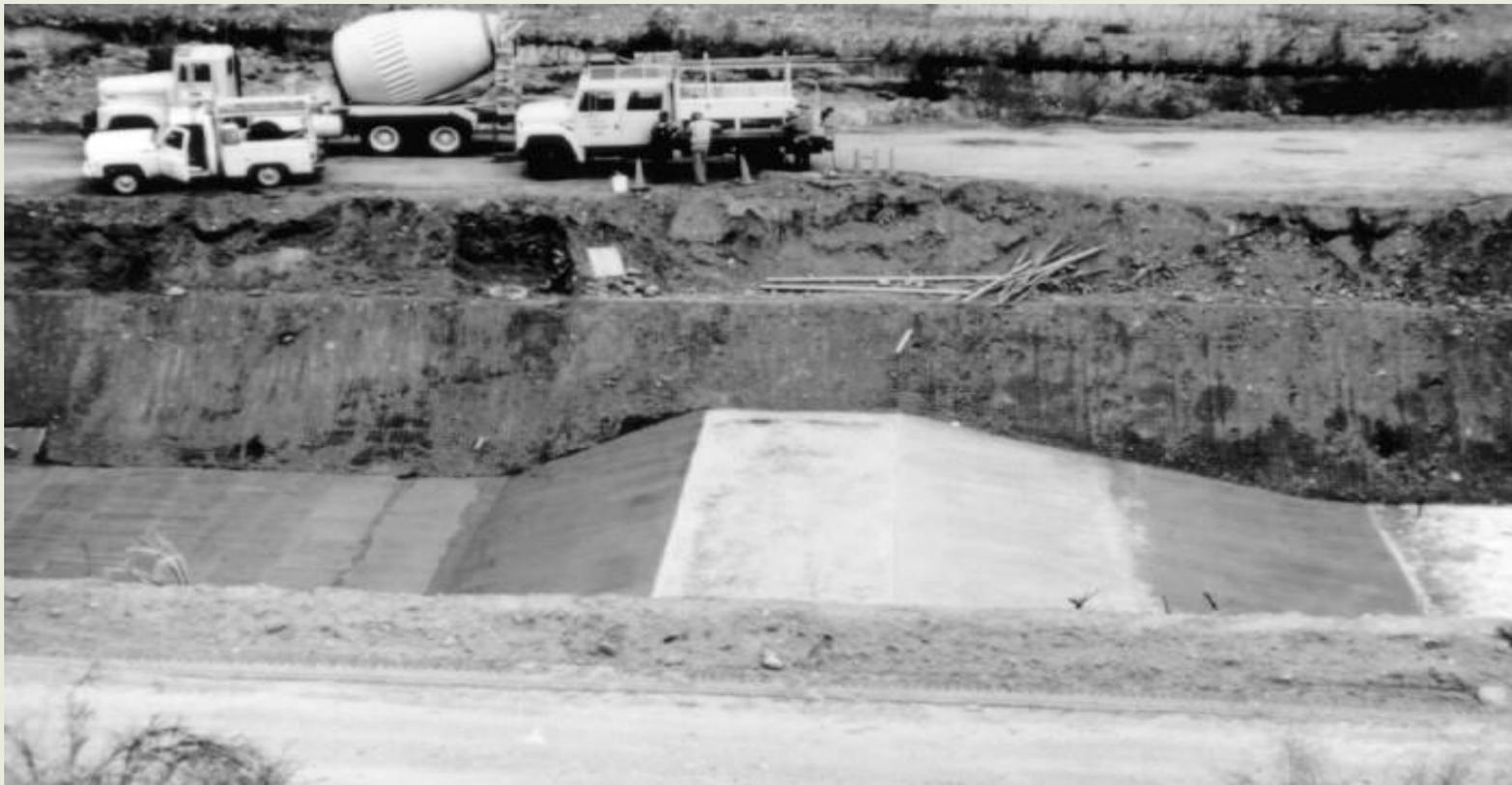
A broad crested weir (BCW) being built. We will be installing BCW's to increase the accuracy of measuring how much water 3 state wildlife areas are receiving.
