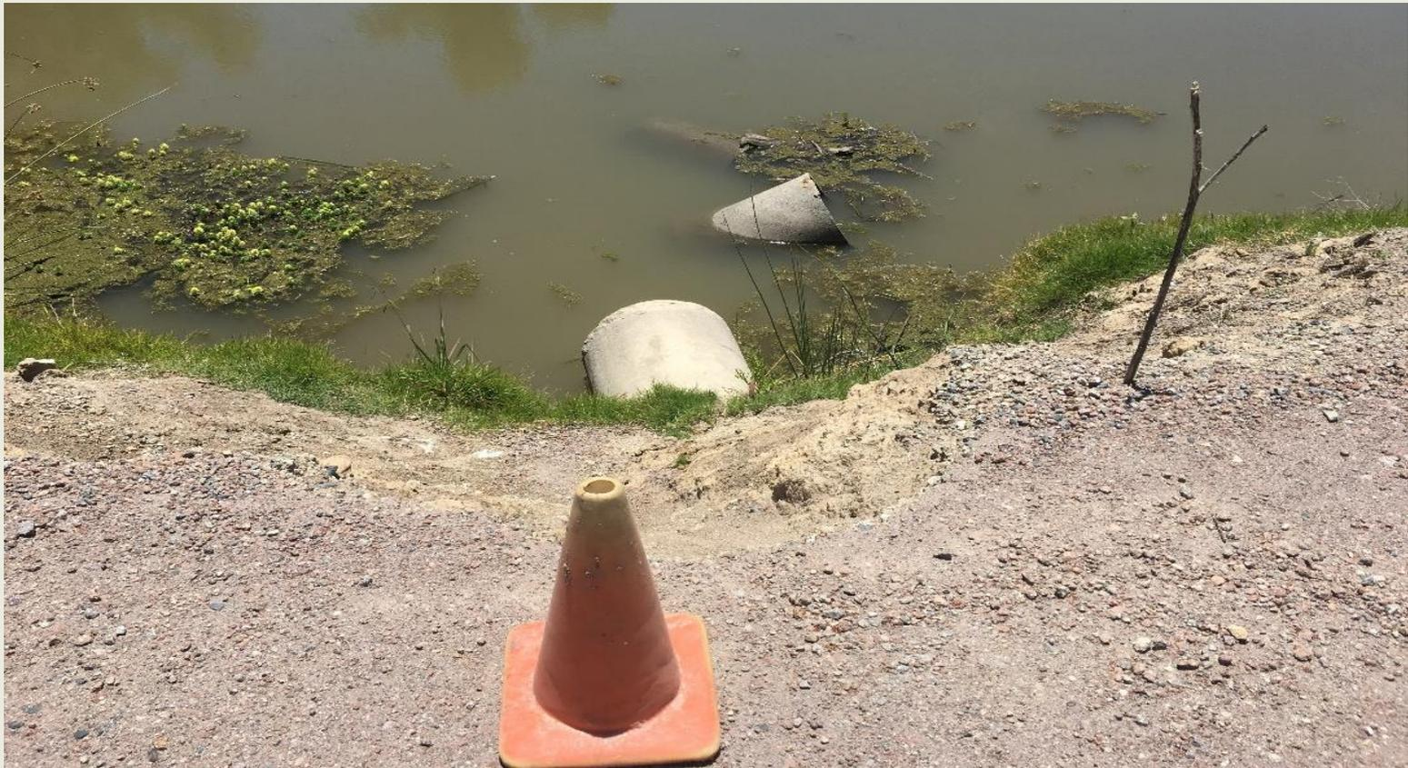
Degraded water control structures will be replaced with new structures to improve water conveyance
