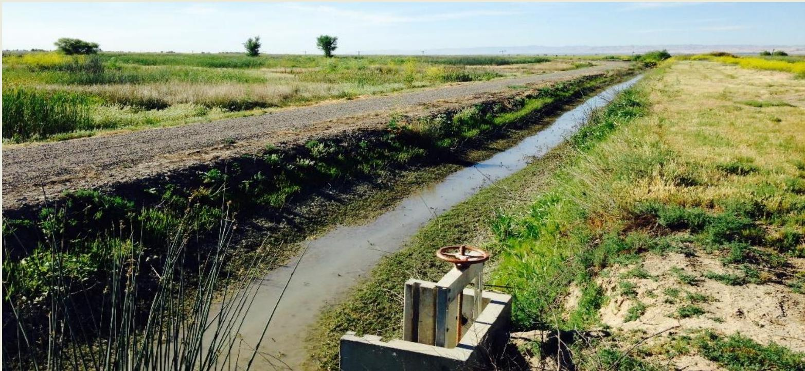
A section of the main delivery ditch bank on the Gadwell Unit will be built up to allow the wildlife area staff to build up head pressure to push water into adjacent units. Currently, water almost floods over the existing ditch bank (left side of picture) when building up head pressure.
