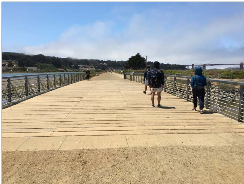
Figure 2. Crissy Field Promenade pedestrian and bicycling bridge in 2017, after the decking boards were rolled over in 2015 as part of this project, and before complete replacement of the decking in 2017.
