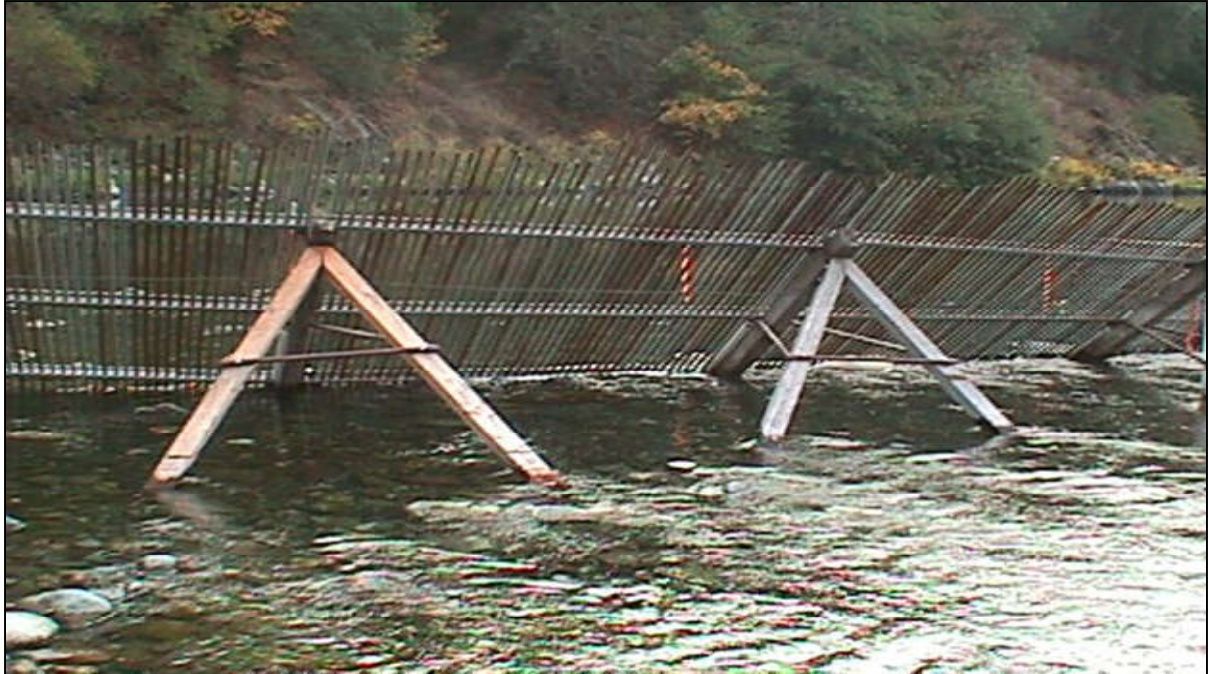
Figure 2. Photograph of Alaskan-style weir, tripods, support channels, and conduit (looking upstream). Picture taken at Willow Creek weir, 2017.
