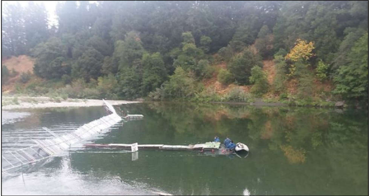
Figure 4. Configuration of Willow Creek weir in 2017. Note the boat gate on the left, with a tunnel leading to the closer of the two traps, and the far side trap mostly submerged.
