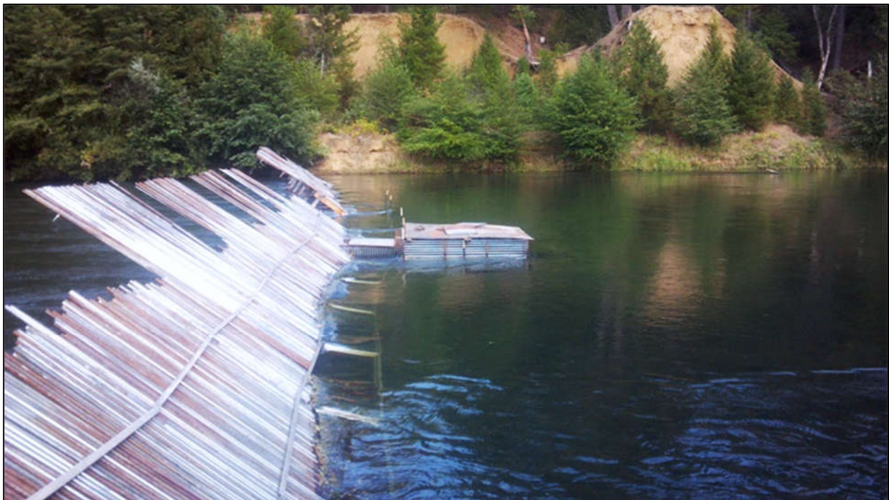
Figure 3. Typical Junction City weir (JCW) configuration. This shows the weir in afternoon "open" mode, with conduit raised and boat gate removed.
