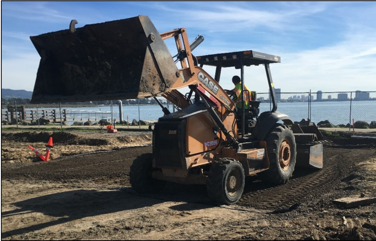
Image 8: South Cove East Parking Lot - Grading and compaction of the existing unconsolidated subsoils atop Bay muds to prepare the base layer for asphalt paving. (Photo by D. Sheils)
