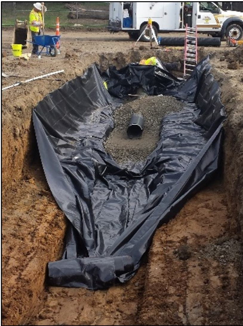
Image 4: Example installation of new storm drain pipes. (Photo by D. Sheils)
