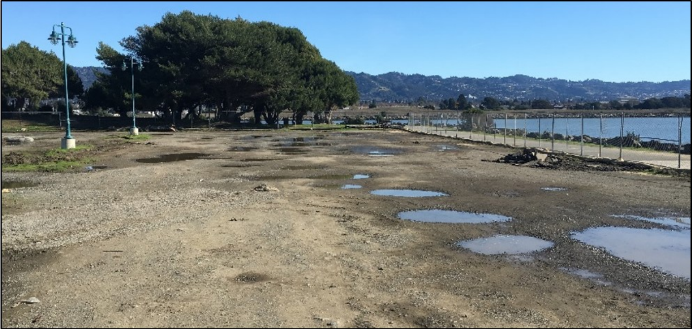
Image 1: South Cove East Parking Lot – Prior to construction. A badly deteriorated gravel parking lot with poor conditions (drainage, striping, pedestrian safety, etc.). (Photo by R. Miller)
