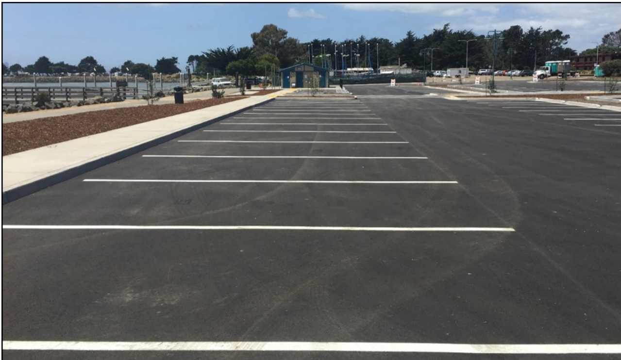
Image 21: South Cove East Parking Lot - After renovation (looking west), there is a newly paved parking lot with new striping, accessible parking and paths of travel, new stormwater bioswales, and a new public restroom. (Photo by D. Sheils)
