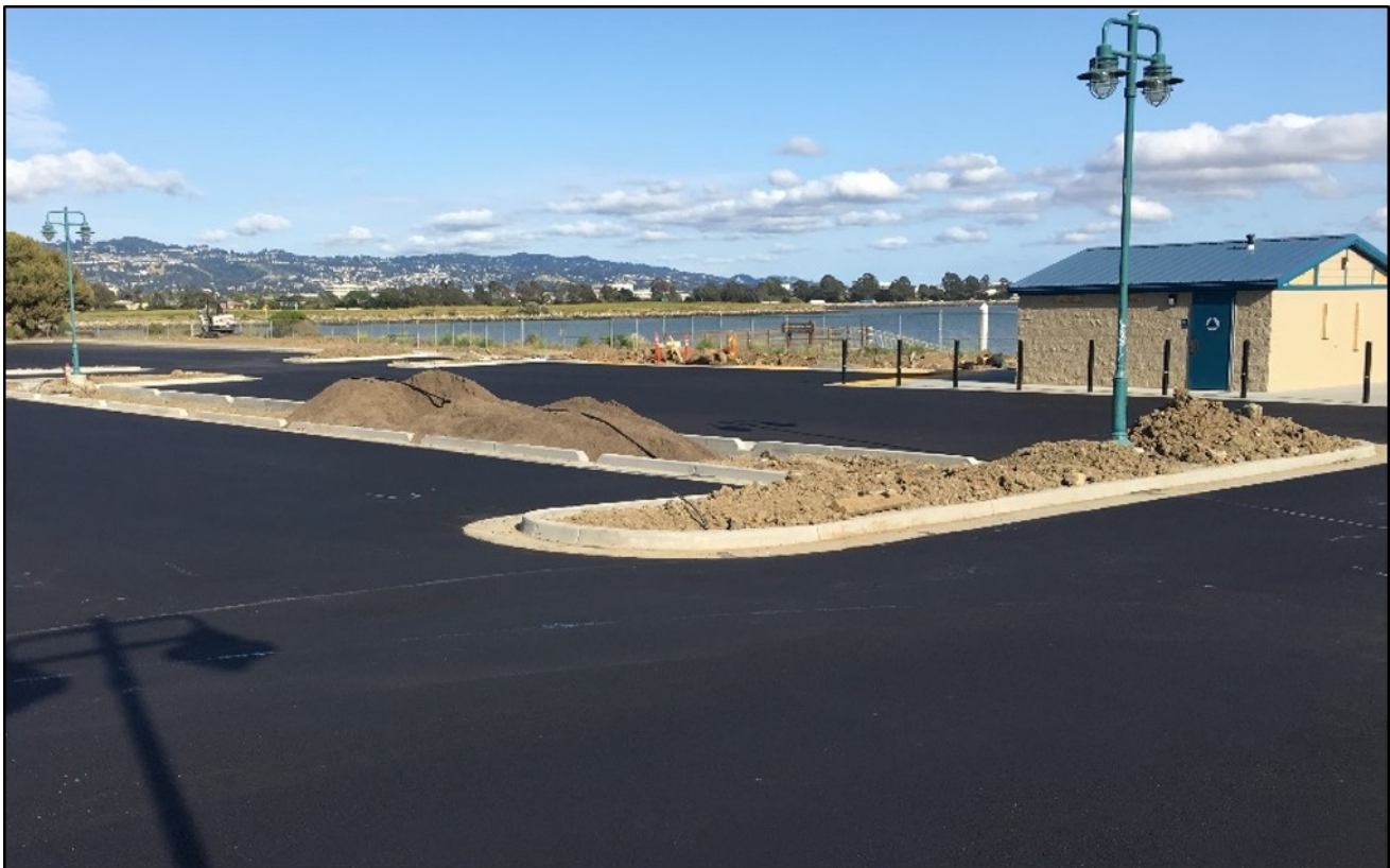
Image 11: South Cove East Parking Lot - The full parking lot was paved in one day. Traffic and ADA striping came later after the asphalt cured. (Photo by D. Sheils)
