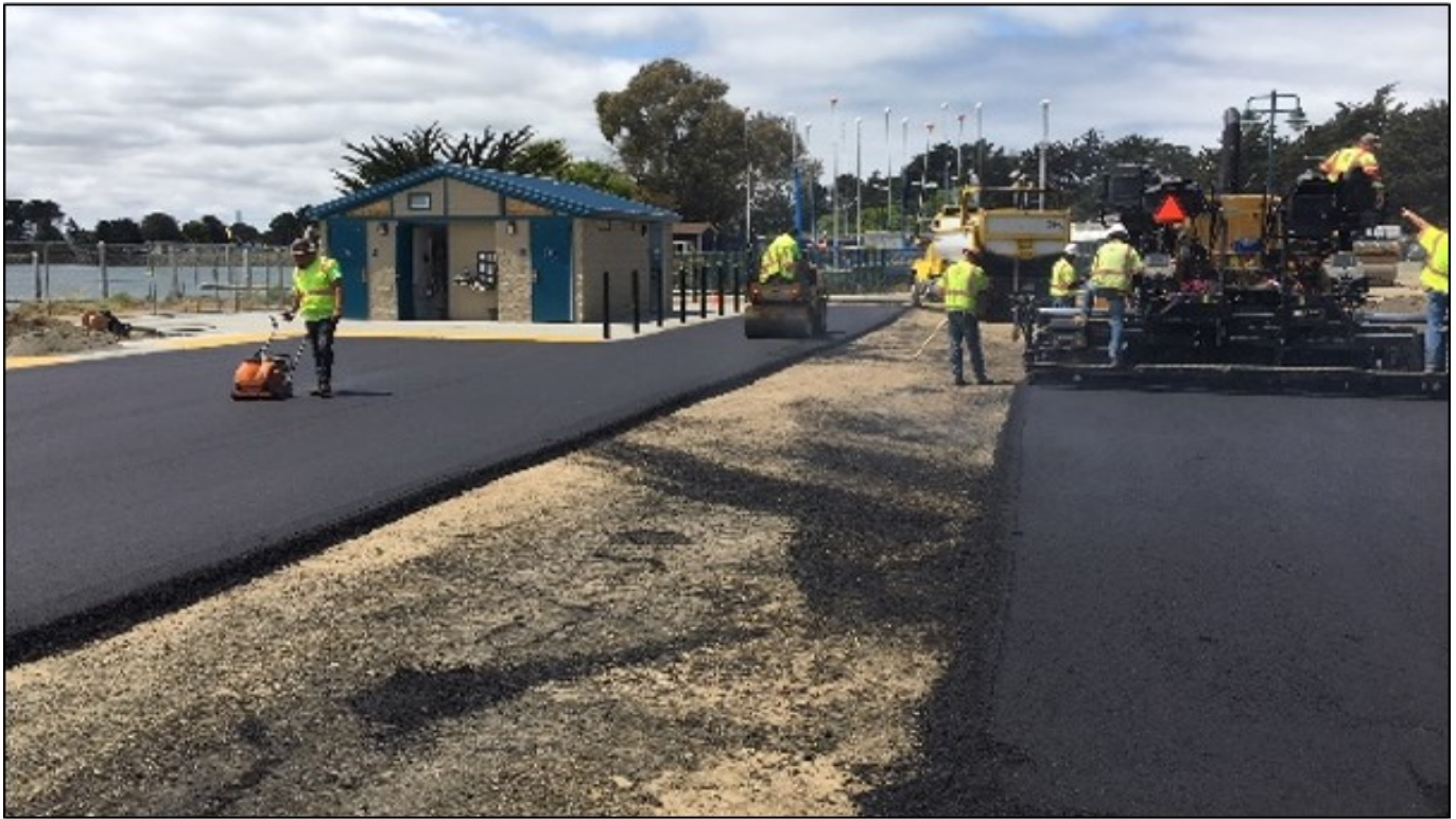
Image 10: South Cove East Parking Lot - New asphalt paving atop the stabilized base layer. (Photo by D. Sheils)
