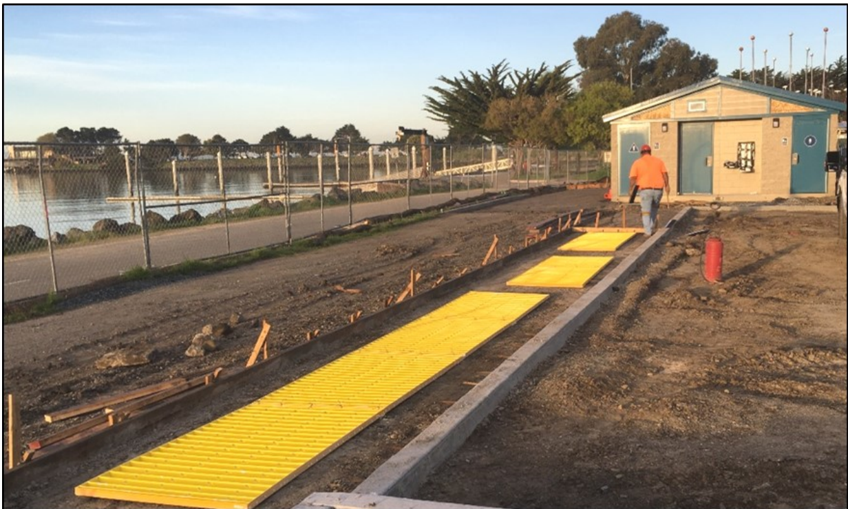
Image 7: South Cove East Parking Lot – Installing truncated dome detectable surfaces for the new accessible concrete sidewalk path of travel from the renovated parking lot to the new public restroom. (Photo by D. Sheils)
