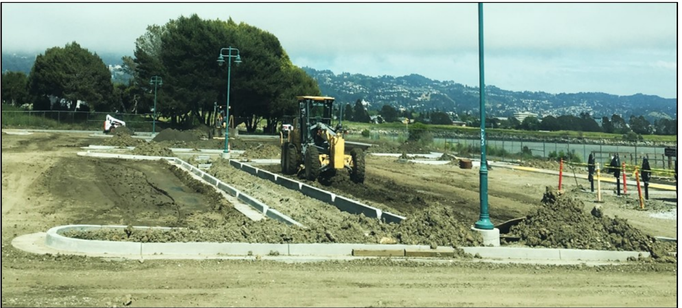
Image 2: South Cove East Parking Lot – Mid-way through construction. Subsoil is being graded and compacted to provide a strong structural base layer for the new asphalt. (Photo by D. Sheils)
