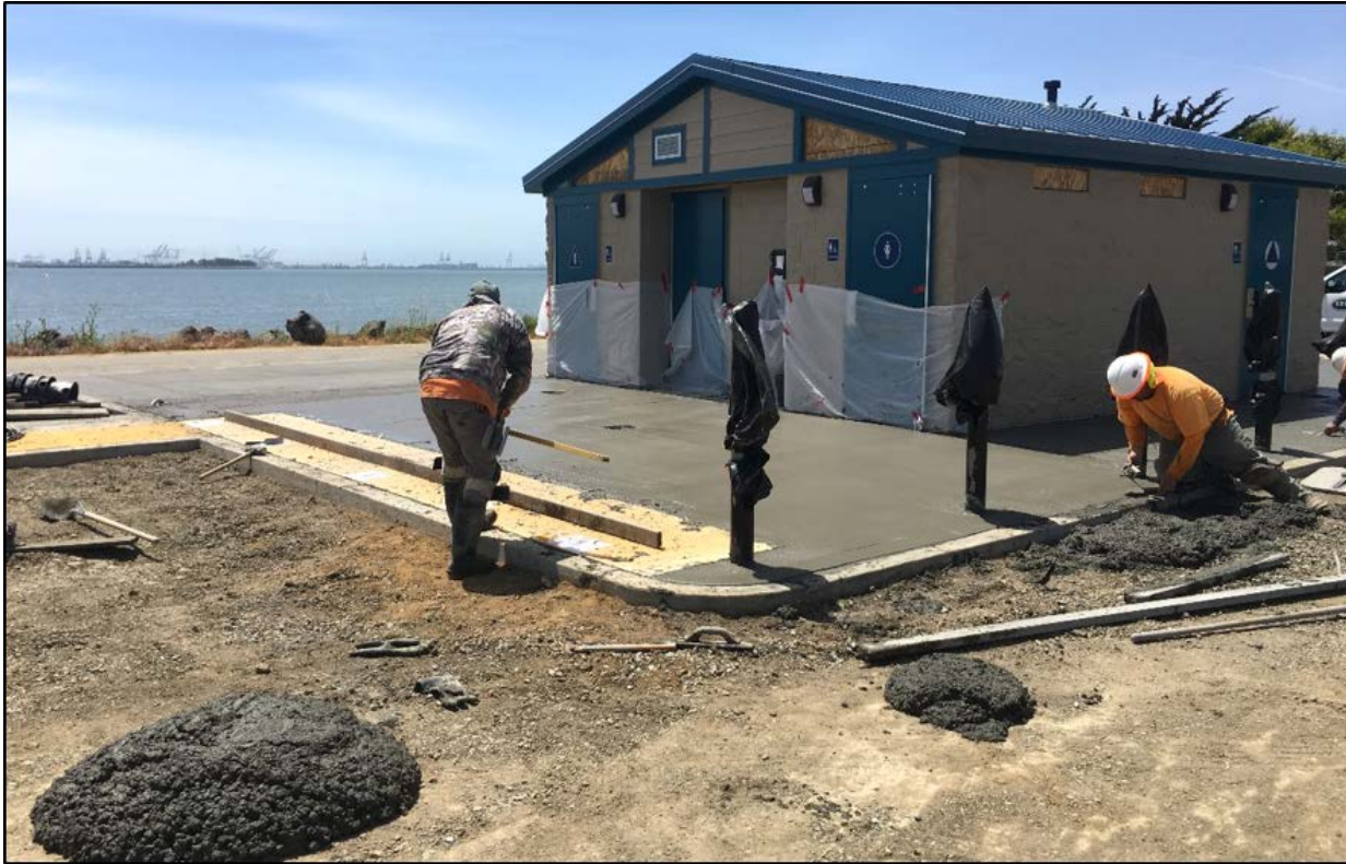
Image 6: South Cove East Parking Lot – Installing the new concrete restroom plaza adjacent to ADA accessible parking slots to provide accessible paths of travel. (Photo by D. Sheils)
