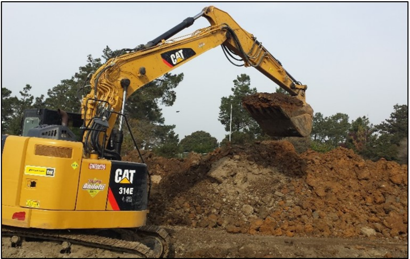
Image 3: South Cove East Parking Lot – Excavating large trenches to install new storm drain pipes and pre-cast storm drain structures to drain new bioswales that remove pollutants from stormwater before it enters the San Francisco Bay. (Photo by D. Sheils)
