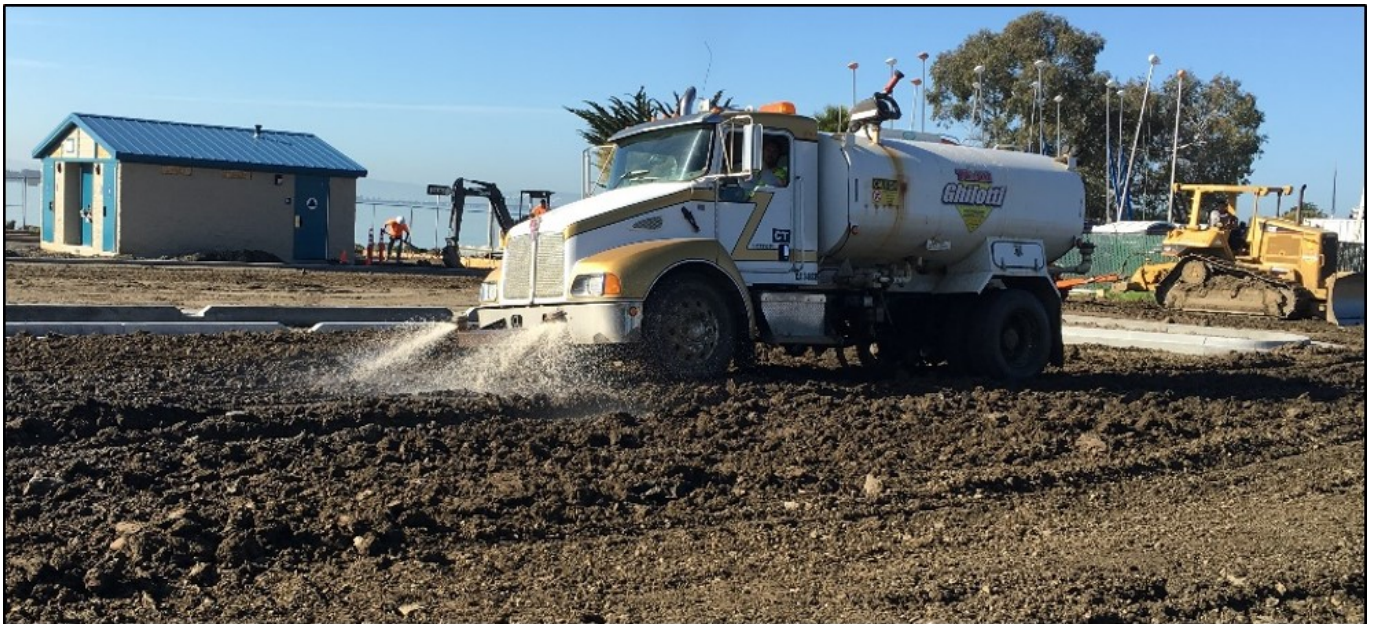
Image 9: South Cove East Parking Lot - Hardening the existing site soils with a soil stabilizer via water truck to create an eighteen inch structural base layer for the top asphalt layer. Re-using the existing soils greatly reduced the need to off-haul soils to the landfill. (Photo by D. Sheils)
