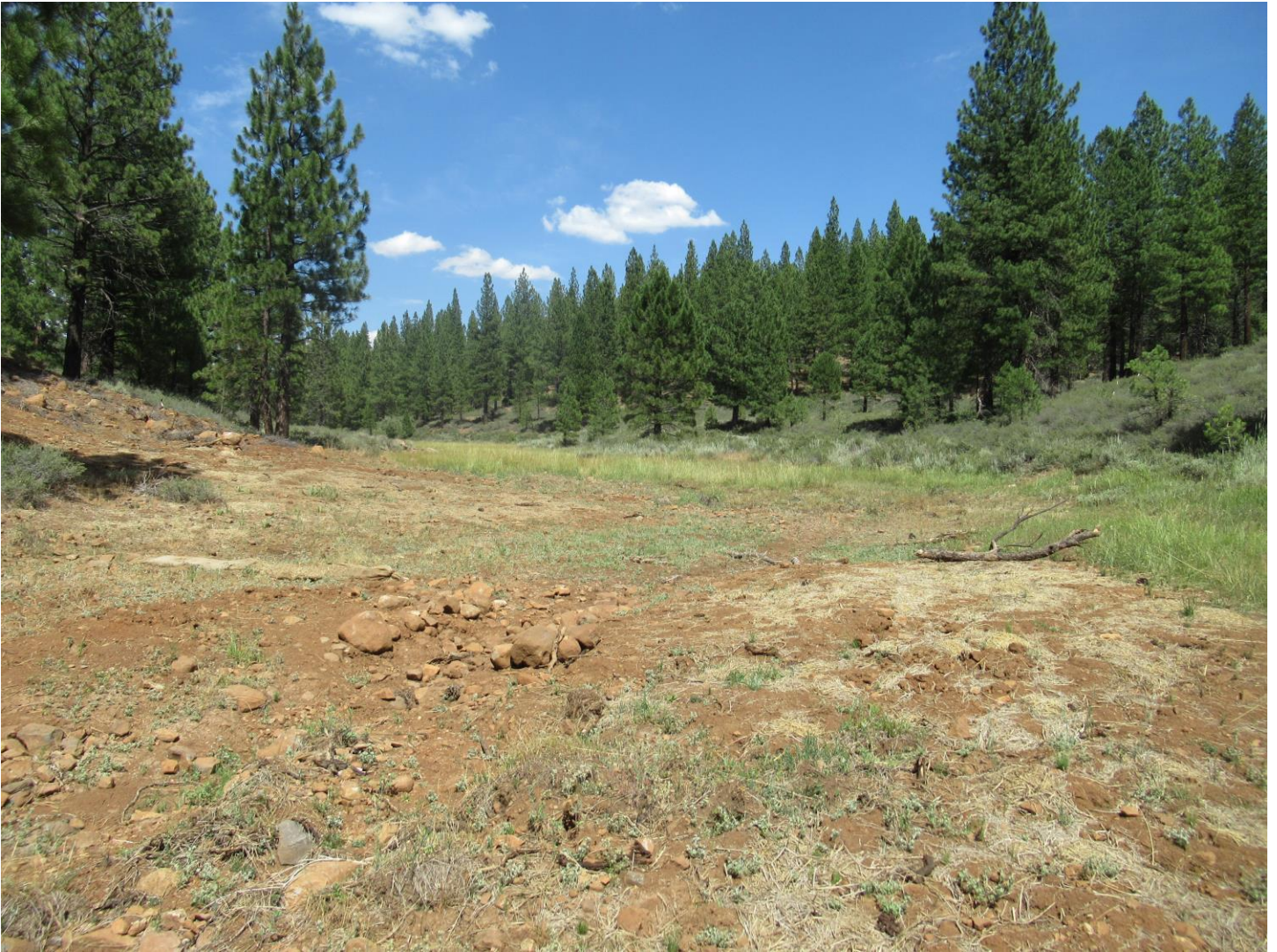
Image 1: Photograph at Site 5 of headcut repair. Prior to project implementation, the headcut was migrating upstream into high quality meadow habitat. The project arrested this erosion.
