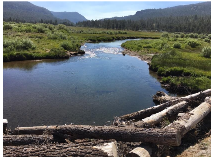
Log crib structure at American River Stream Bank Project Site
