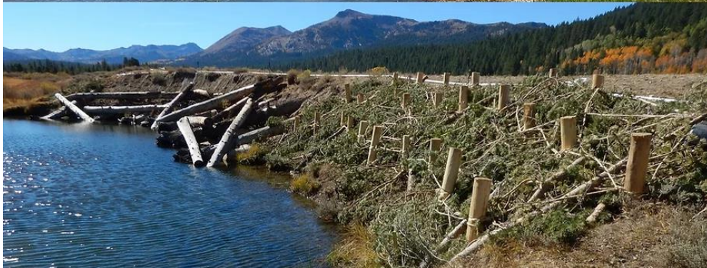
Project Site 2 before (above) and after construction (below) - updates were needed to divert stream energy from scouring behind the 2015 log crib structure so slash was installed at the ends of reach to add stability.
