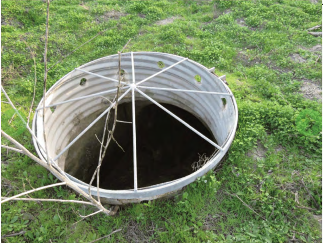
One of the illegal drains – demonstrating how the rainwater would enter the structure and be sent out to sea – instead of nourishing the wetlands. (Photo by Jonathan Coffin)
