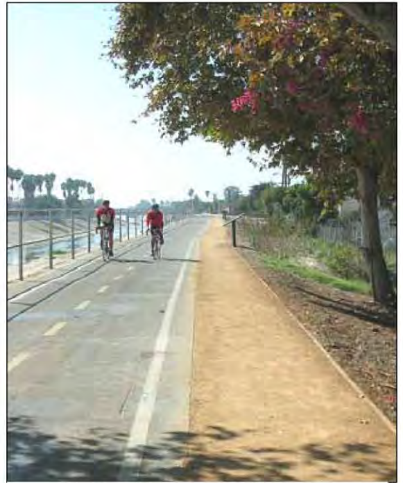
New pedestrian walkway, with interpretive signs.
