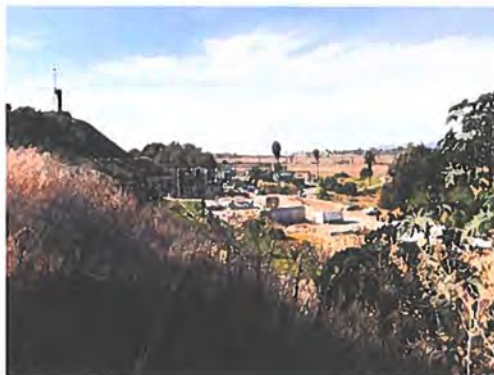
SOCALGAS GAS STORAGE FIELD TANK FARM CULVER BLVD, PLAYA DEL REY, CA
