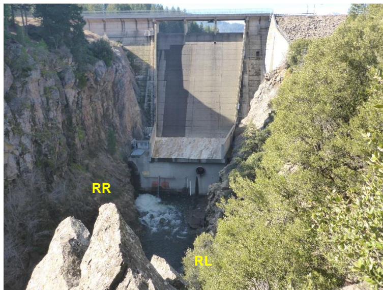
Box Canyon Dam
