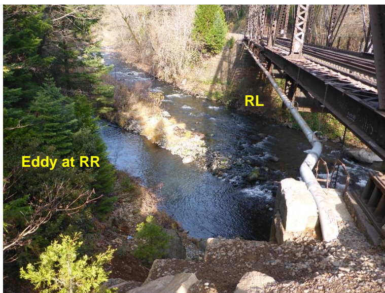
Straight Across at Rail Bridge
