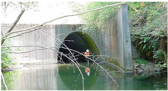
Figure 55. Partial culvert barrier where Highway 101 crosses Rattlesnake Creek in the Eastern Subbasin.
