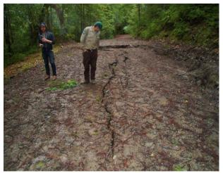
Figure 26. Example of legacy road failure in the SF Eel River Basin.
