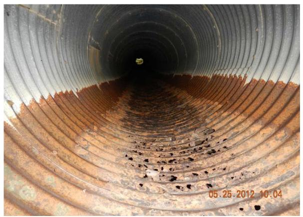
Figure 56. Failing culvert on Dinner Creek, tributary to China Creek in the Western Subbasin (photo courtesy of Scott Bauer, CDFW).
