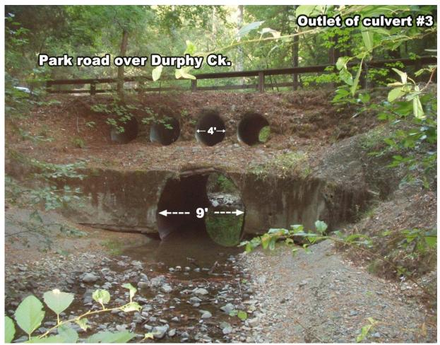
Figure 55. One of two partial culvert barriers located on Durphy Creek.
