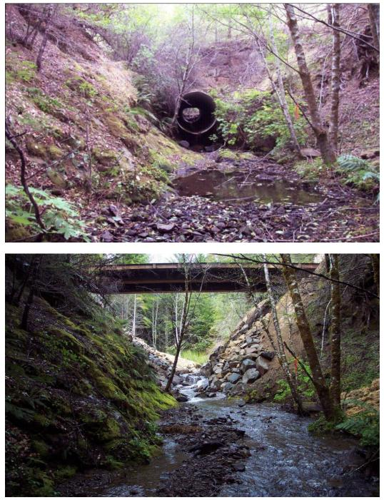
*Figure 57. Example of upslope watershed restoration project in Hollow Tree Creek before (above) and after (below) treatment (Pacific Watershed Associates 2010).*
