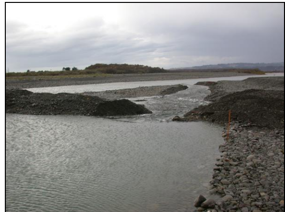
Figure 12. Excavated channel with exclusion culverts (top) looking upstream and looking downstream with culverts removed (bottom) to allow fish passage into Van Duzen River at flows of ~160 cfs.
