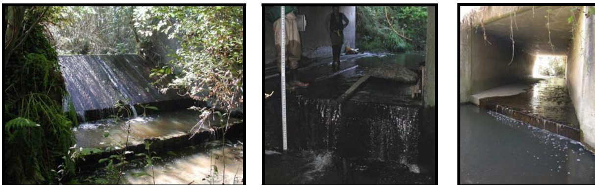
Figure 34. Examples of fish passage barriers in the upland Salt River tributaries.
