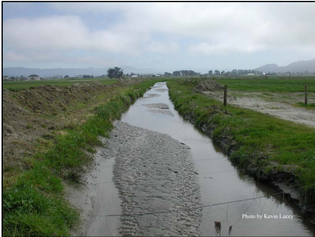
Figure 17. Reas Creek upstream of Meridian Road on December 3rd, 2004.
