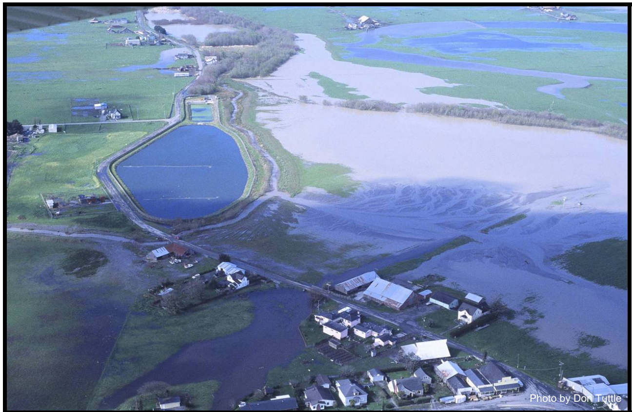
Figure 21. Westward aerial view of the Ferndale waste water treatment plant during February 2004. The ponded area on the right is known as Lake Vevoda. Francis Creek flows around the settling pond, Arlynda Corners is in the foreground.
