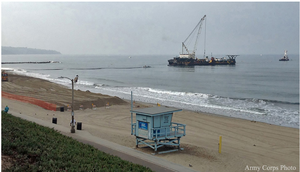
Figure 2. Beach sand replenishment between Topaz Jetty and Redondo Pier, CA, USA on 5 October 2012.
