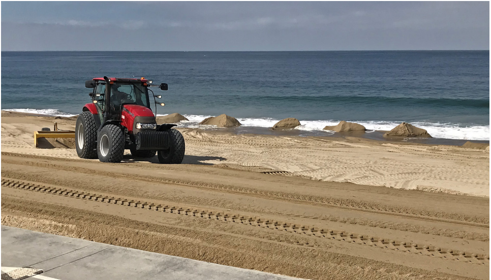
Figure 3. Spreading dump truck-deposited sand at Redondo Beach with rubber-tired equipment.
