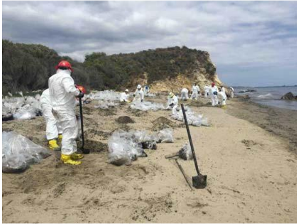
Figure 11. Manual removal of oil and oily material from sandy shorelines. Stranded kelp, also known as wrack, was one material that was removed from shorelines.
