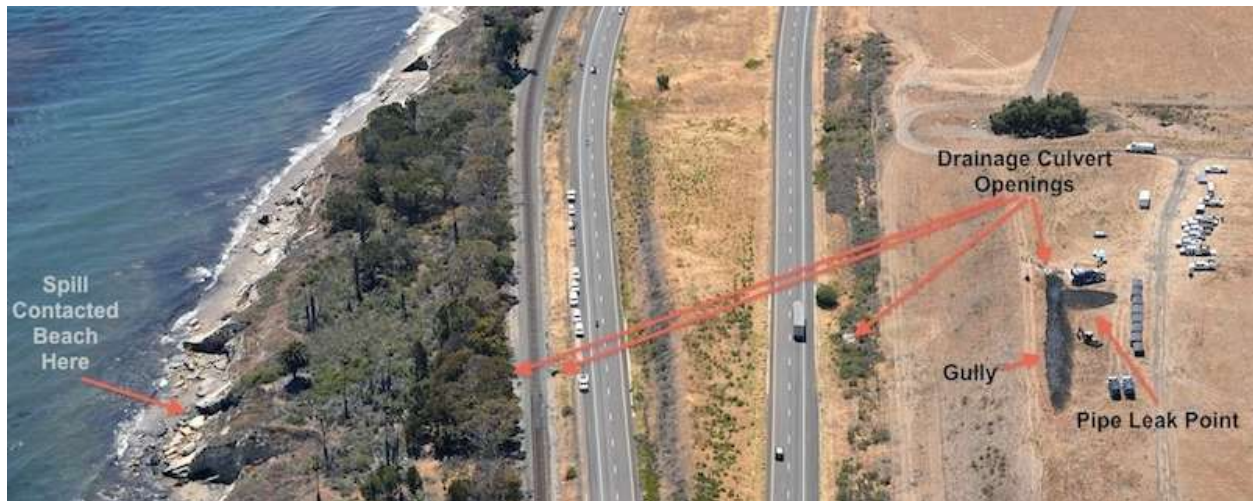
Figure 1. Flow path of the Line 901 pipeline rupture into culverts under Highway 101 and railroad tracks and ultimately into the Pacific Ocean at Refugio State Beach. Credit: John Wiley ( http://flickr.com/jw4pix )
