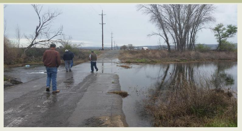
Dye Creek running over Shasta Boulevard after a winter storm event. The current culverts are insufficient to handle the average amount of water flow.
