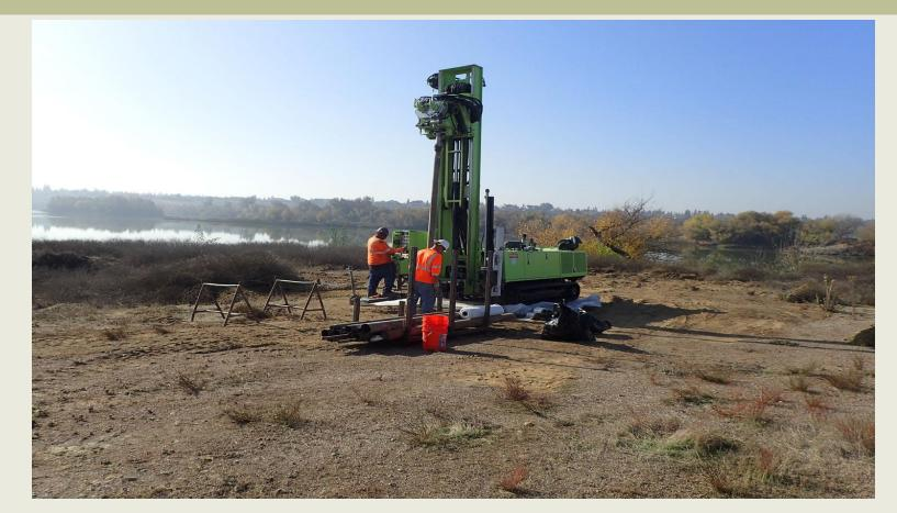
Pond berm drilling and substrate sampling in 2017 during preliminary study phase
