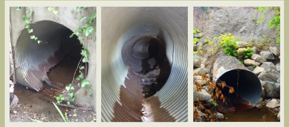
Photo 1: Upstream inlet of culvert Photo 2: Interior of culvert showing damage to corrugated metal pipe Photo 3: Downstream outlet of culvert
