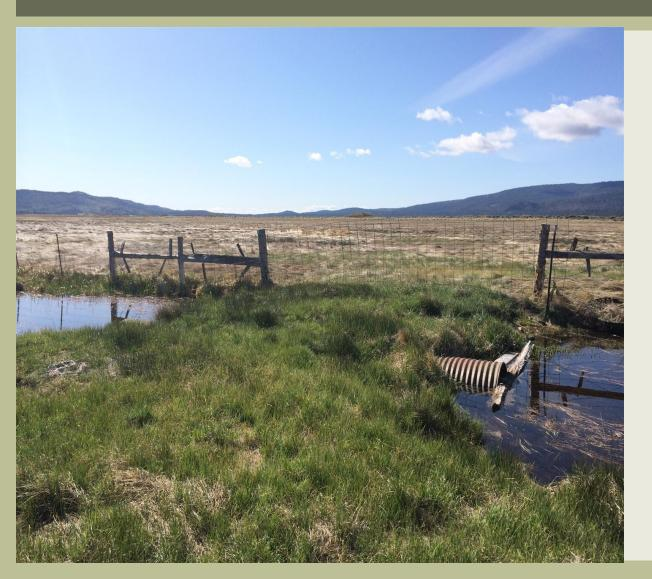
Failing corrugated metal pipe culverts, set at incorrect elevations will be replaced with HDPE pipe
