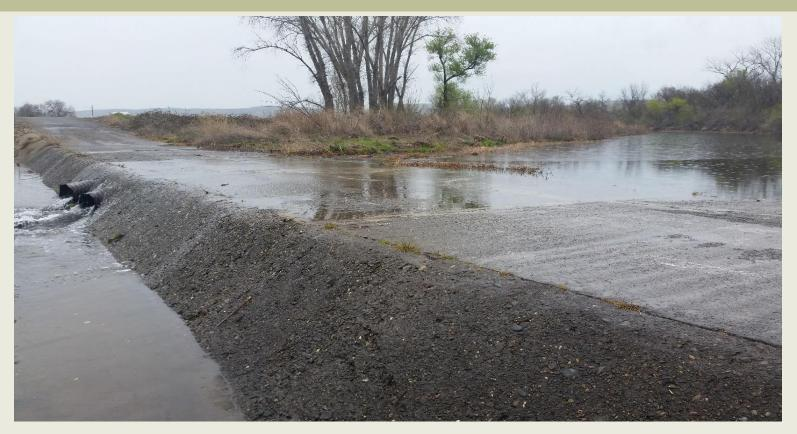
The current low water crossing with its undersized 12inch diameter culverts has filled with sediment and is impeding fish passage.
