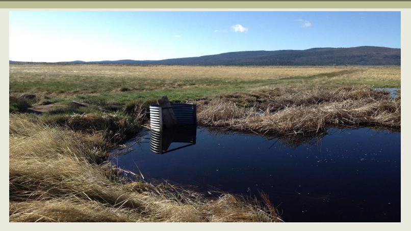
Old corrugated metal half-round risers will be replaced with new cast concrete weirs
