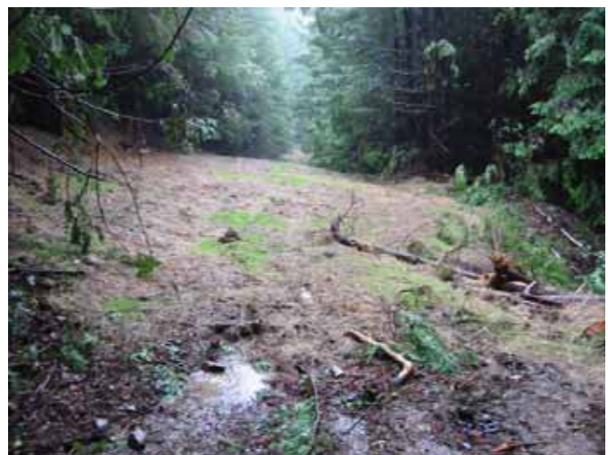
Figure 39. Abandoned road re-contoured to natural slope.
