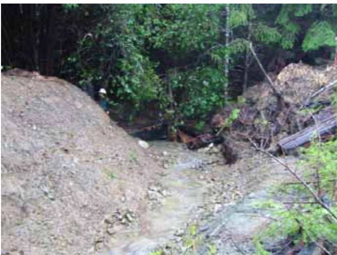
Figure 37. Legacy watercourse crossing removal.
