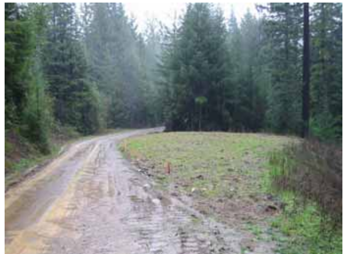
Figure 38. Reclaimed landing on mainline road.
