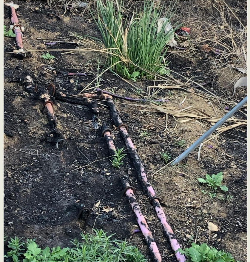
Fire Damaged Bio-swale And Irrigation Lines
