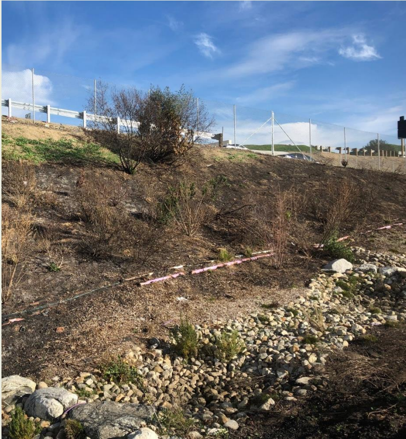
Fire Damaged Bio-swale And Irrigation Lines
