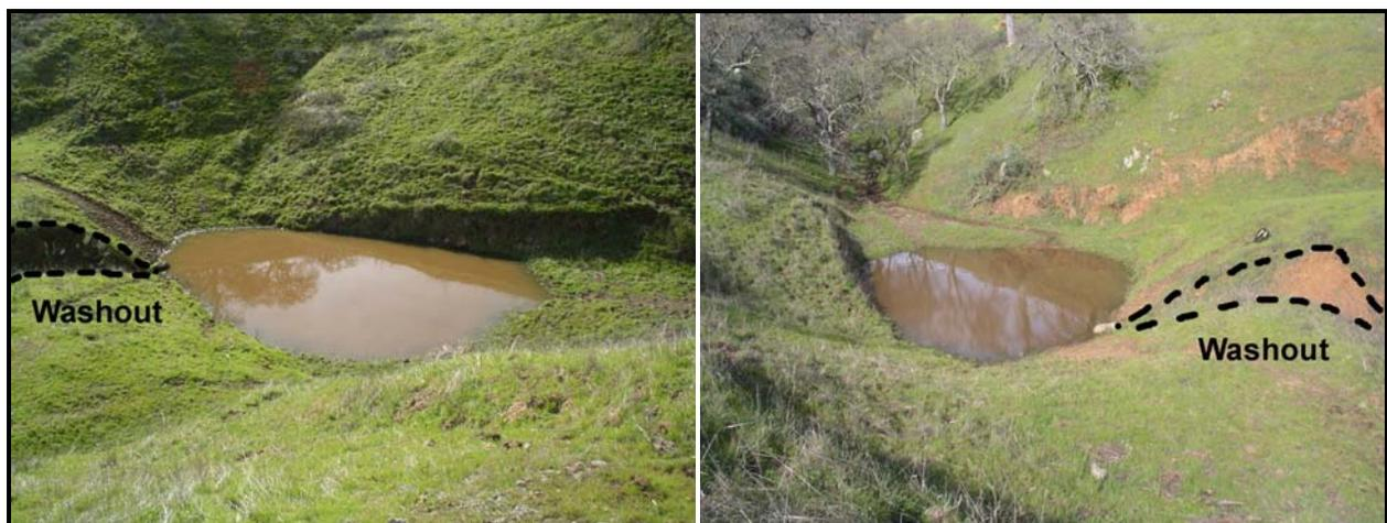
Figure 3. Upper Cottonwood Creek Wildlife Area berm erosion at Big Bully Gully while viewing pond from east side (at left) and from southwestern side (at right), 2006.
