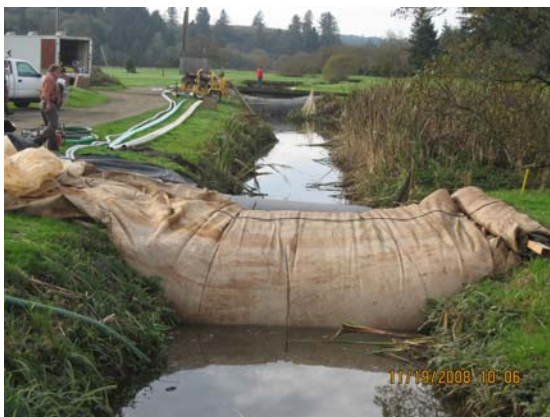
Figure 3. Inflatable dam in place on upstream end of 17 th hole pond (left). Pumps used to drain pond (right).
