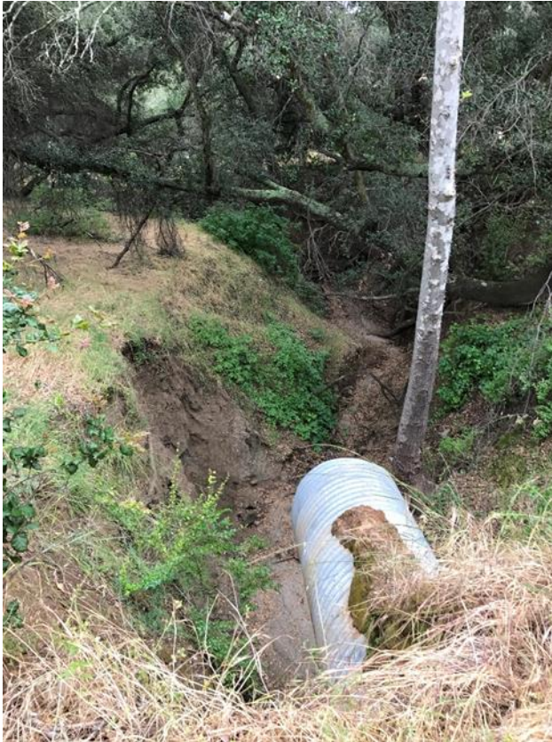
Culvert washout spring 2017, photo by T. Stewart
