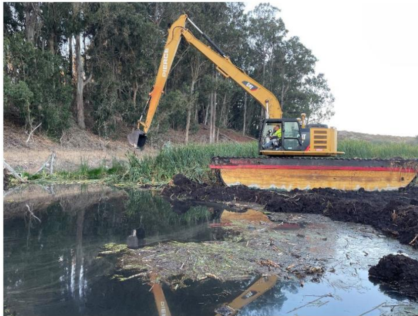
Aquatic excavator removing sediment and vegetation from Black Lake.
