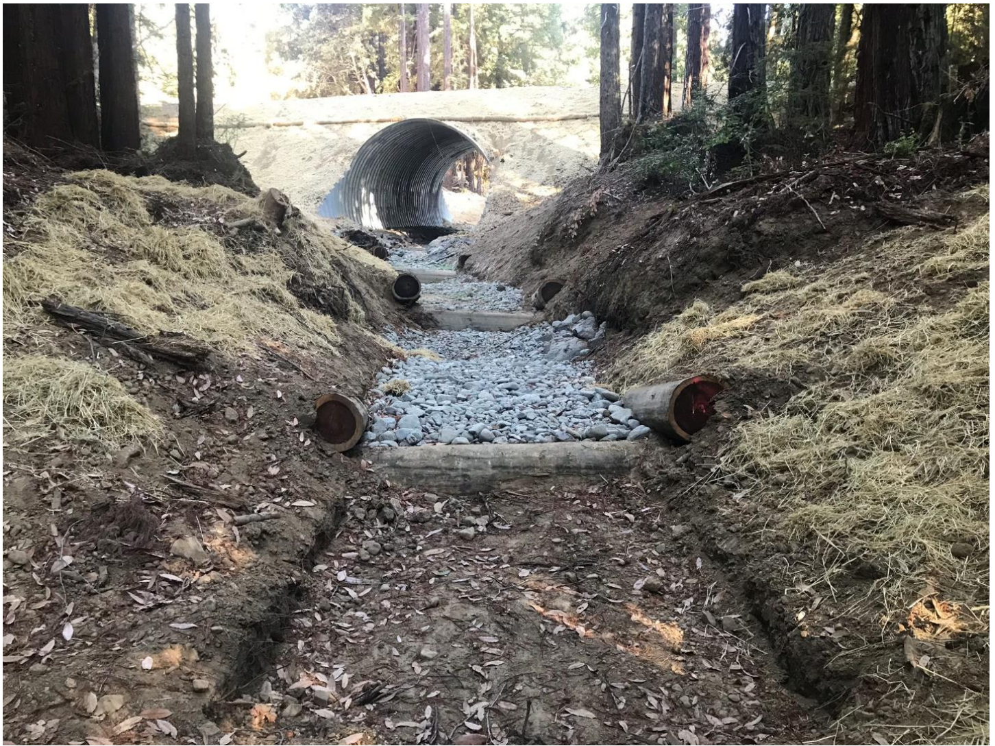
Image 7: Log steps, photo taken at downstream project end, looking upstream.
