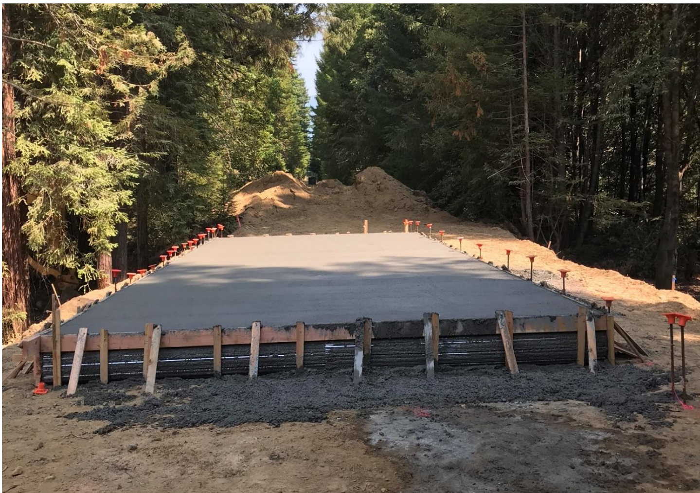
Image 5: Concrete pad placed as structural support on rail bed.
