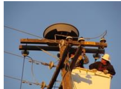
Installation of Osprey Nesting Platform
