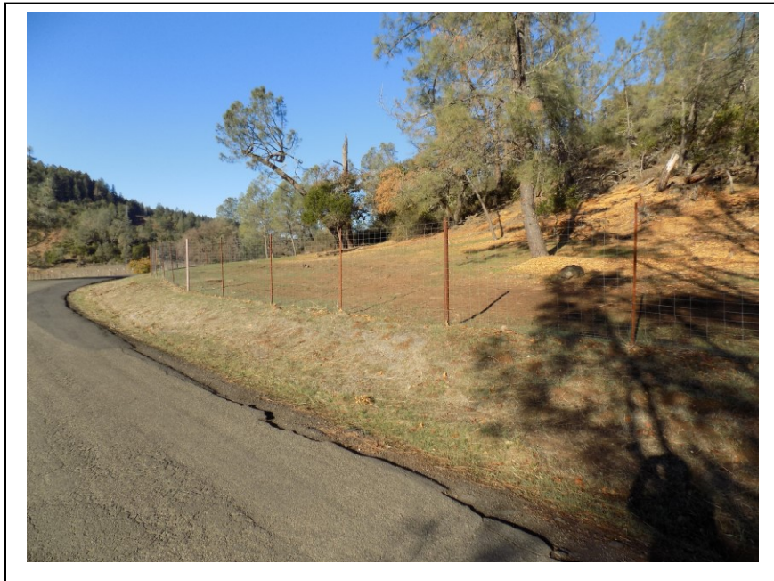
North side of Conn Valley Road recently cleared, scoured and fenced
