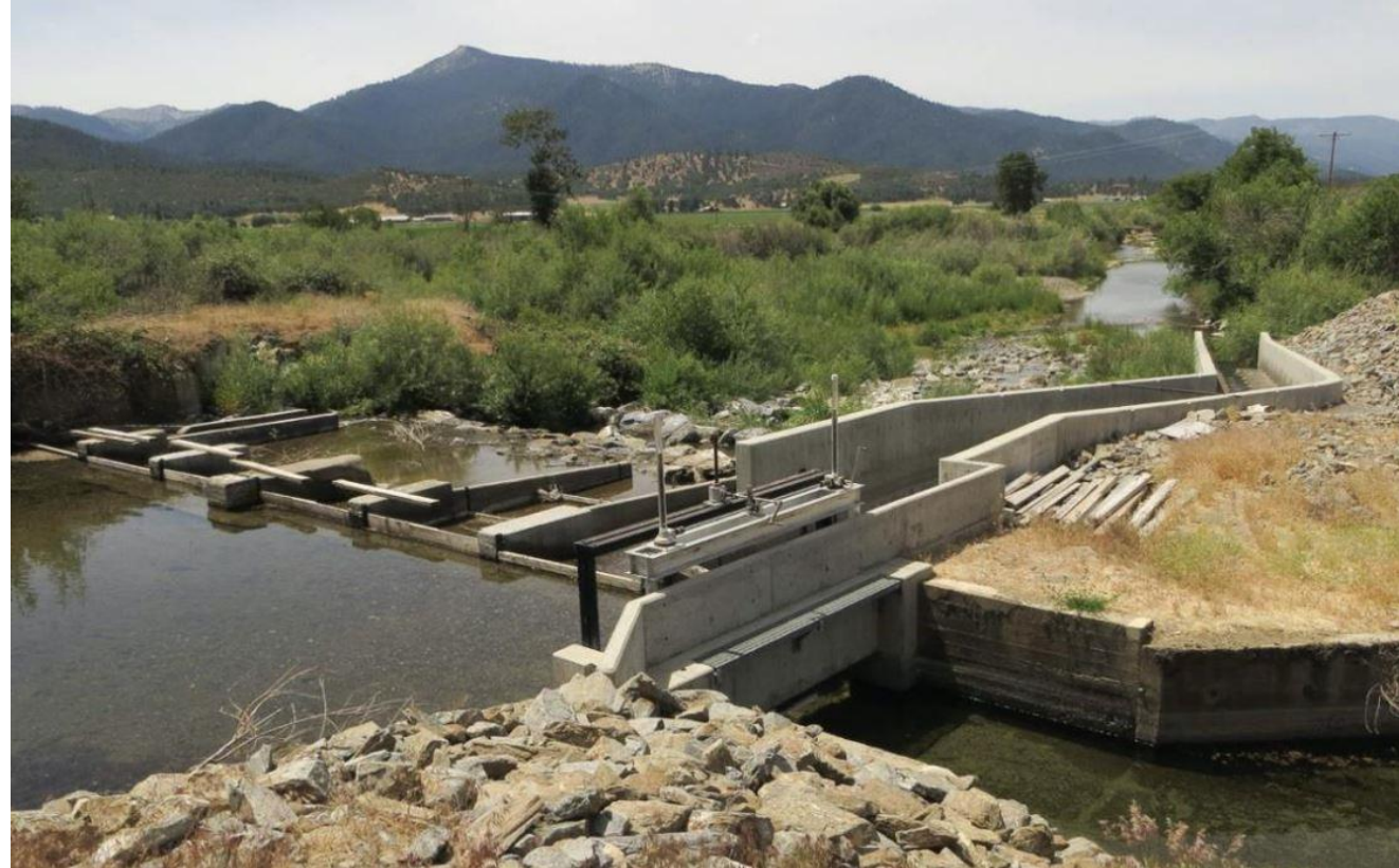
Young's Point diversion structure and fish ladder Credit: Siskiyou Land Trust
