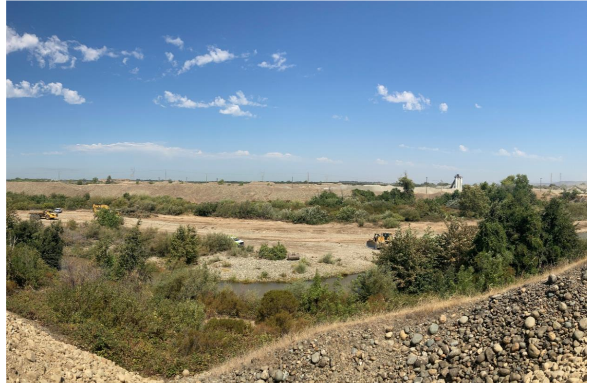
View from the Middle Training Wall. Photo credit: CBEC Eco Engineering (April Sawyer)
