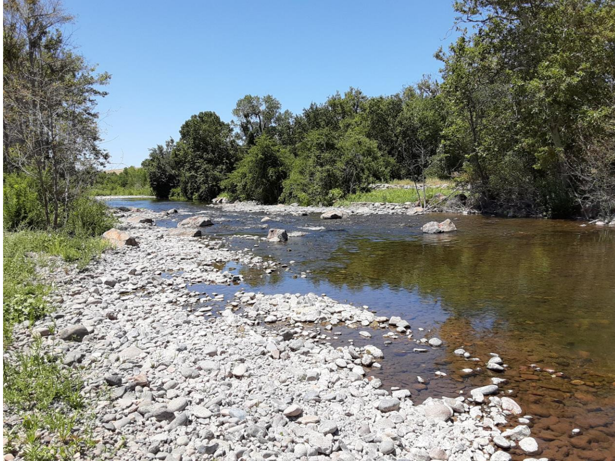
Looking downstream at the Deer Creek Irrigation District roughened rock ramp Credit: Ben Cook, Trout Unlimited.
