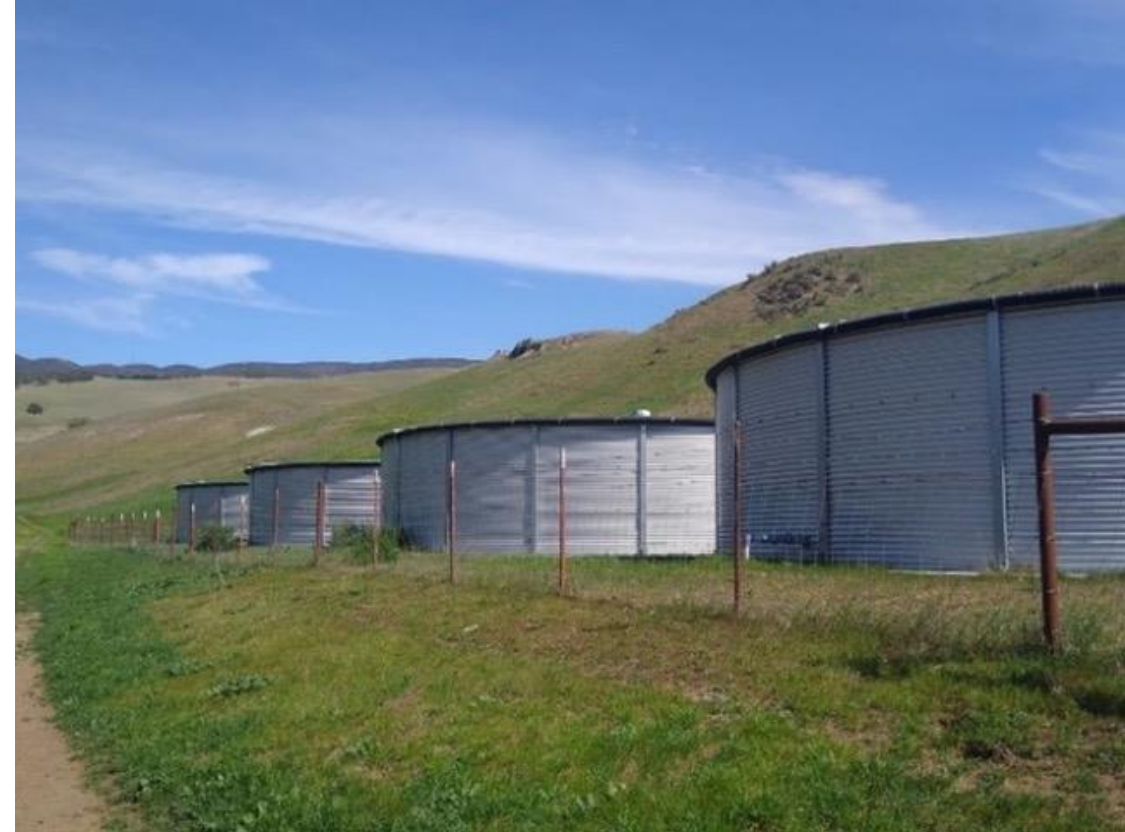
Existing tanks at Escuela Ranch. Credit: Aleksandra Wydzga
