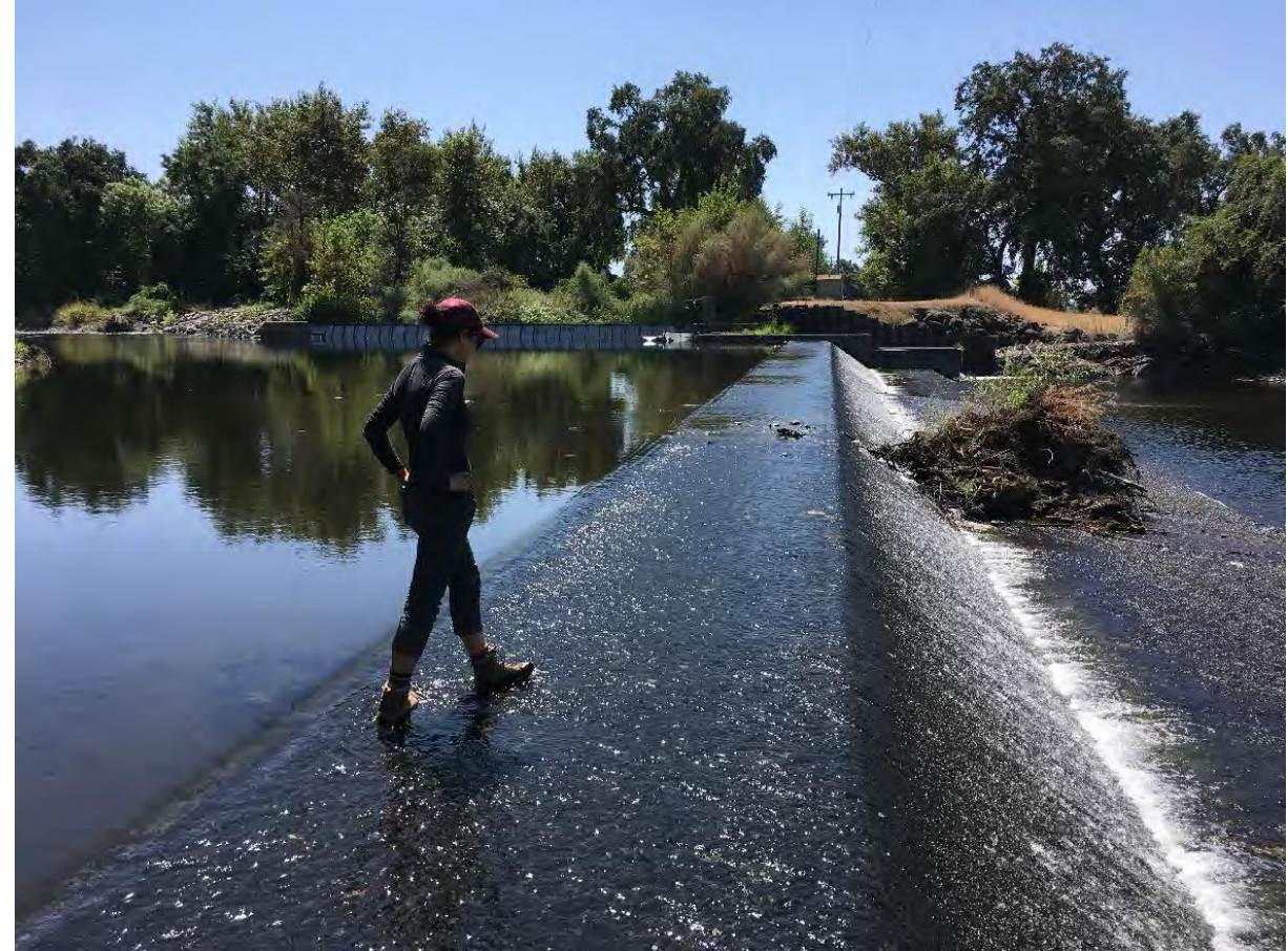
Stanford-Vina Ranch Irrigation Company dam Credit: Ben Cook, Trout Unlimited.
