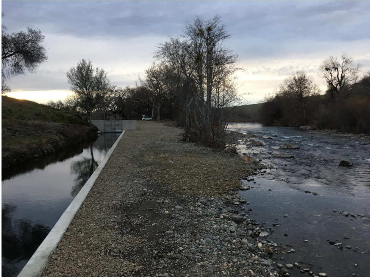
DCID diversion on the left and Deer Creek on the right Credit: Ben Cook, Trout Unlimited
