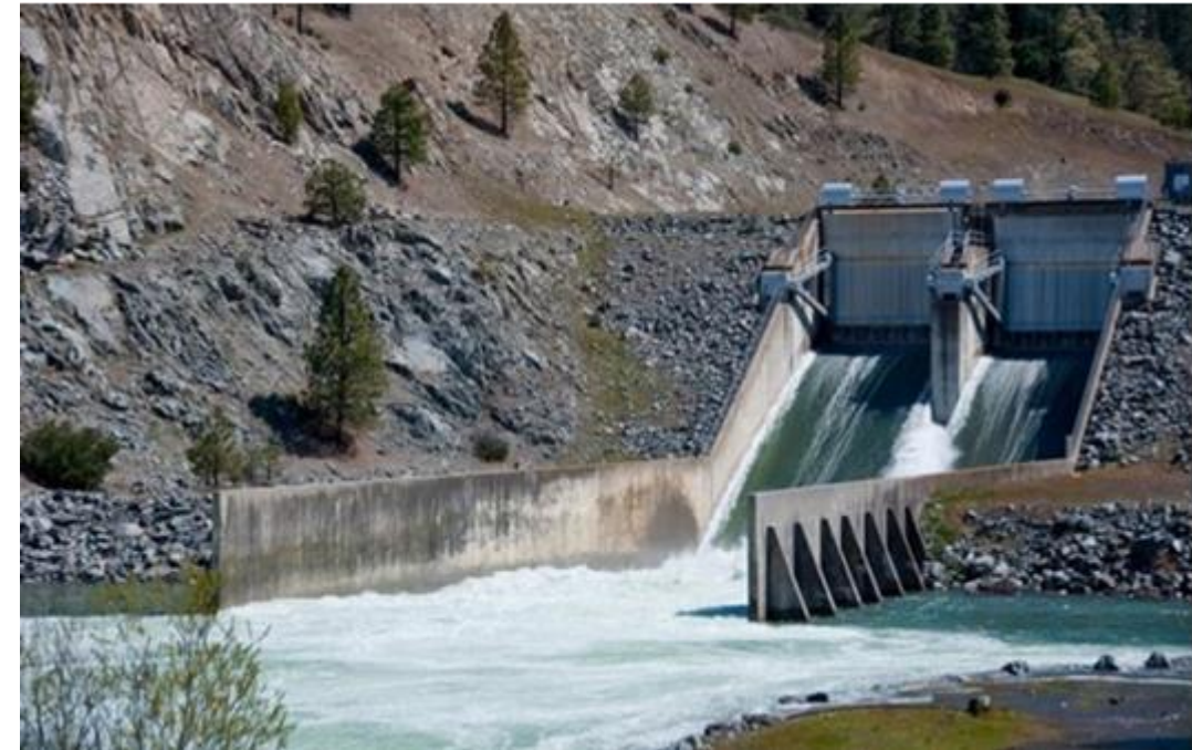
Lewiston Dam provides downstream releases to Trinity River and diverts water to Whiskeytown Lake through the Clear Creek tunnel. Credit: Trinity County Chamber of Commerce
