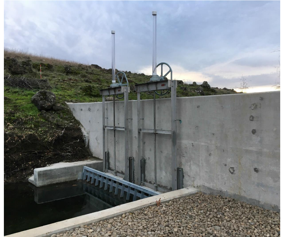
DCID diversion headwall Credit: Ben Cook, Trout Unlimited
