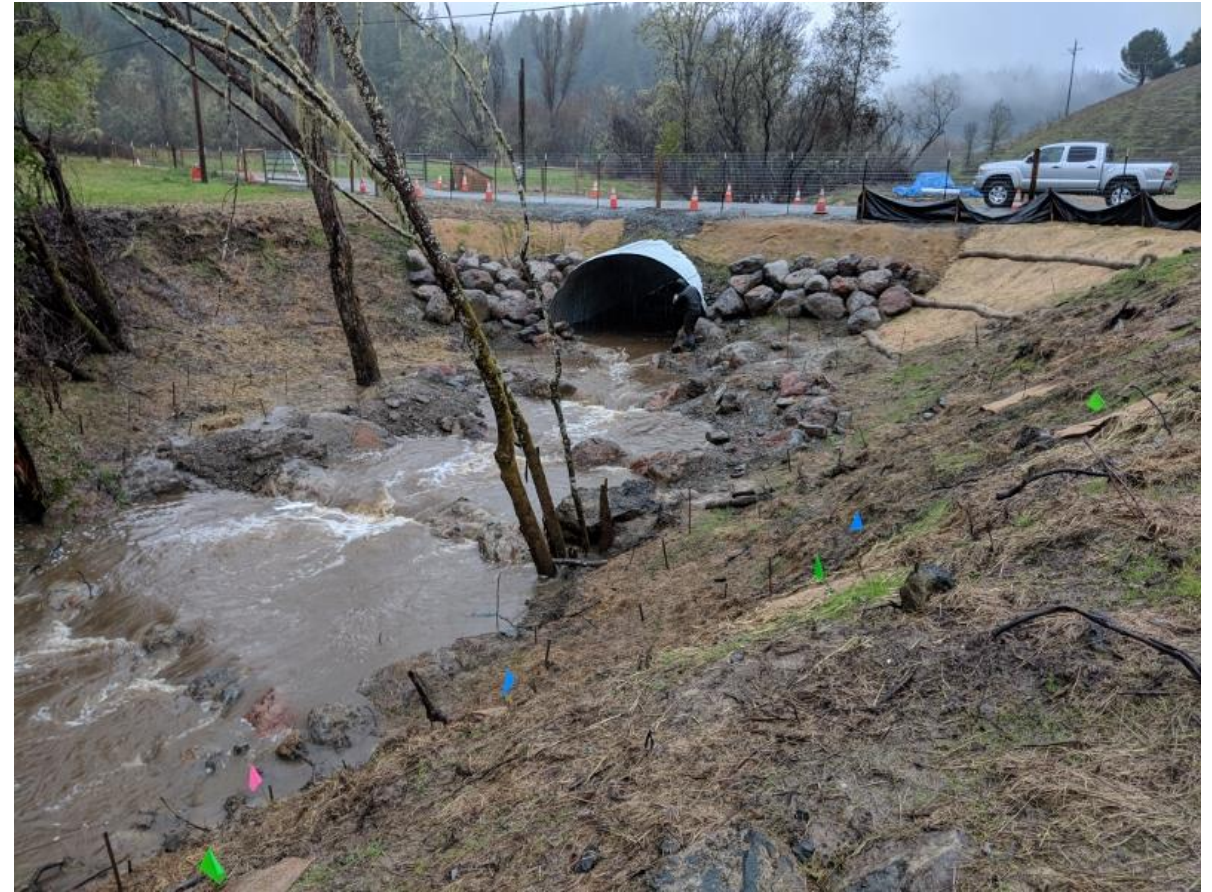
Culvert replacement, January 2018 Credit: John Green, Gold Ridge RCD
