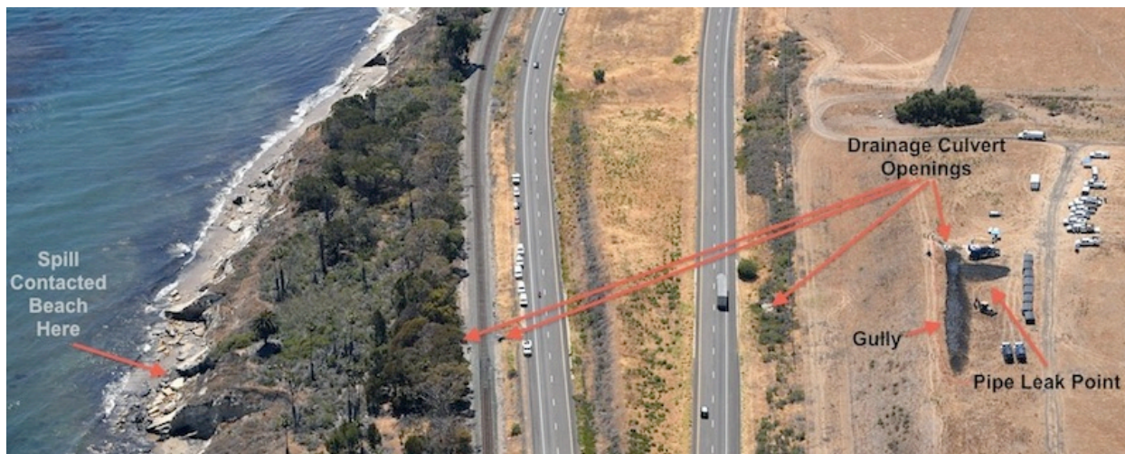
Figure 1. Flow path of the Line 901 pipeline rupture into culverts under Highway 101 and railroad tracks and ultimately into the Pacific Ocean at Refugio State Beach. Credit: John Wiley ( http://flickr.com/jw4pix )
