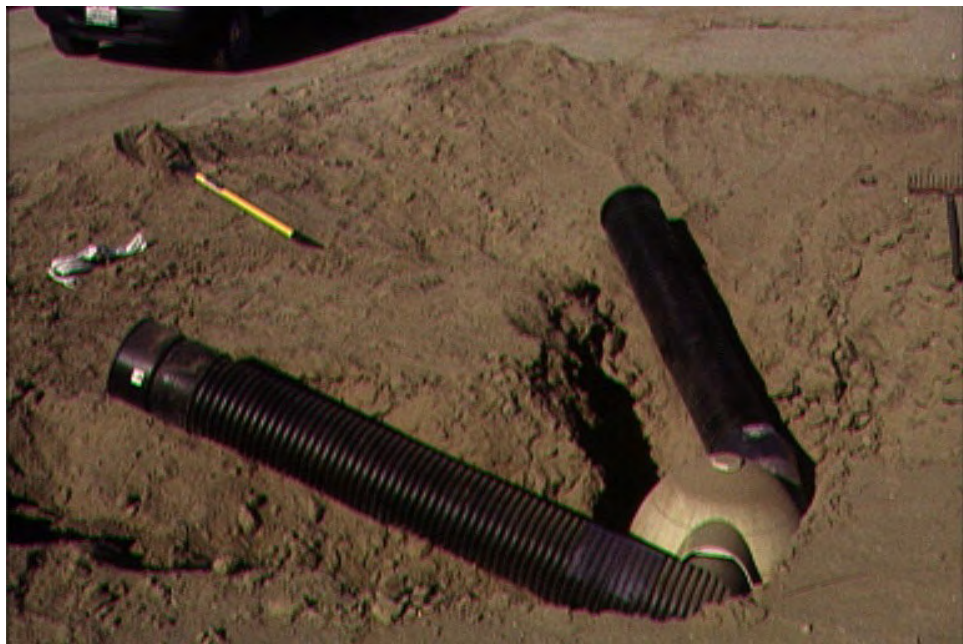
Figure 6. A HDPE two-entrance chambered den with a dogloo chamber being installed for San Joaquin kit foxes in Bakersfield, CA.
