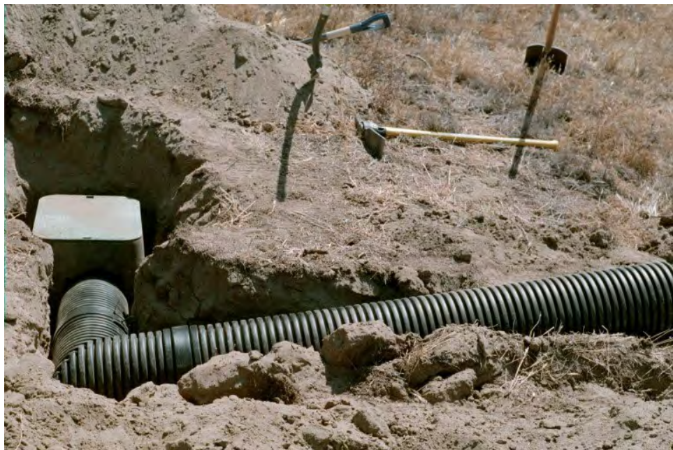
Figure 5. A HDPE one-entrance chambered den with an irrigation box chamber being installed for San Joaquin kit foxes in Bakersfield, CA.
