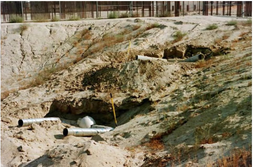
Figure 7. An artificial den complex being installed for San Joaquin kit foxes in Bakersfield, CA. A concrete two-entrance non-chambered subsurface den is being installed on the upper slope and a metal two-entrance chambered den with a dogloo chamber is being installed on the lower slope. A surface den also was installed on the flat ground above the other dens.
