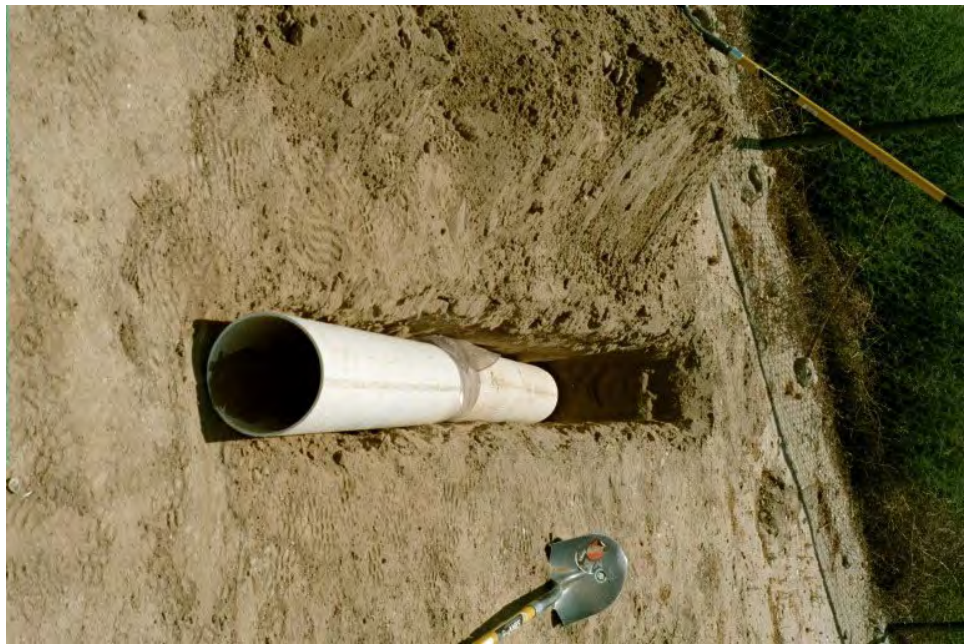
Figure 3. A PVC one-entrance subterranean den being installed for San Joaquin kit foxes in Bakersfield, CA.
