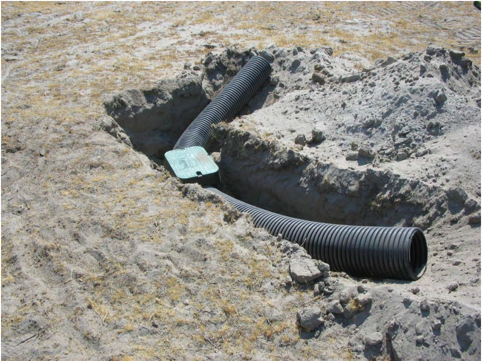
Figure 10. Recommended artificial den design for San Joaquin kit foxes: single-walled HDPE two-entrance chambered den with an irrigation valve box for the chamber.
