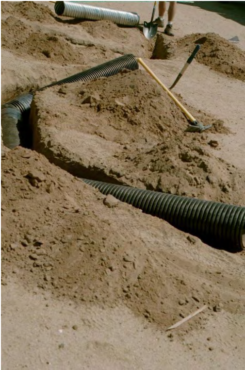
Figure 4. A HDPE two-entrance subterranean den being installed for San Joaquin kit foxes in Bakersfield, CA.
