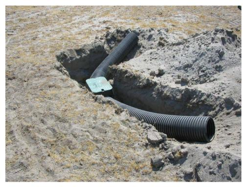
Figure 10. Recommended artificial den design for San Joaquin kit foxes: single-walled HDPE two-entrance chambered den with an irrigation valve box for the chamber.
