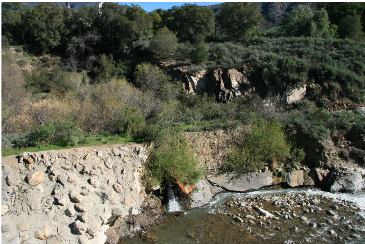
Fig. 18. Northeast of the Culvert Seep Area (foreground), the Thomas Aquinas Oil Pool is in the upper left quadrant of the photo and may be recognized as the light straw-colored vegetation behind the concreted rock rip-rap bank protection. The damaged culvert and soil bank downstream of the rip-rap were heavily eroded by the Jan. 2005 storms. (Photo taken 26 Feb. 2008).
