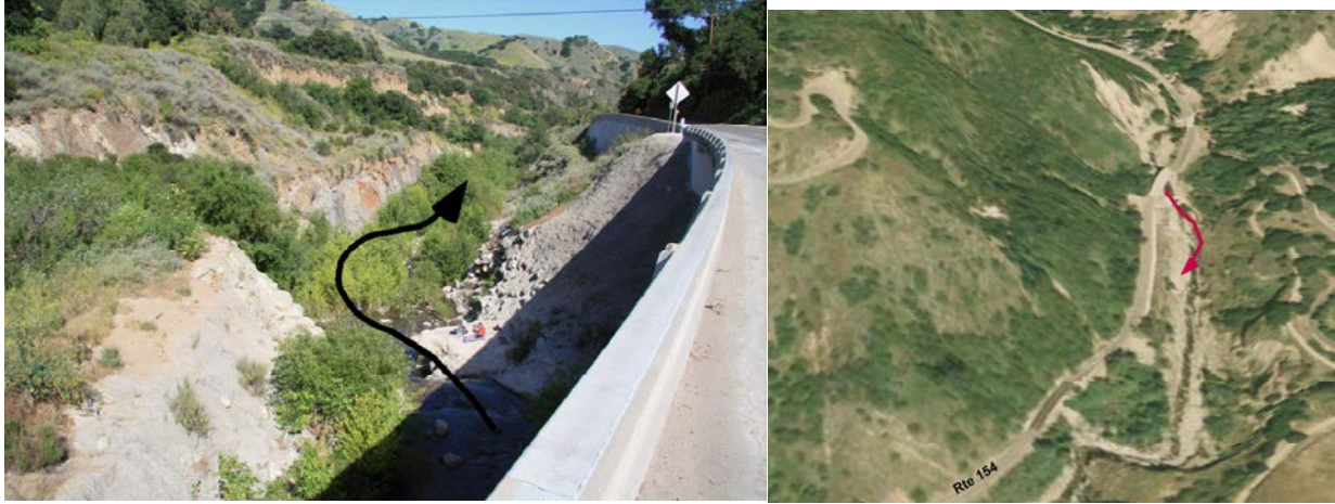
Fig 37. Left. East-southeast-looking photo from the Hwy 150 bridge showing the channel alignment is directed toward the North bank. The upstream end of Thomas Aquinas Oil Pool lies behind the rip-rap to the left. Most of the North bank is unprotected. Right. East-Northeast looking Google Earth overview of valley showing proposed stream water flow during storms.
