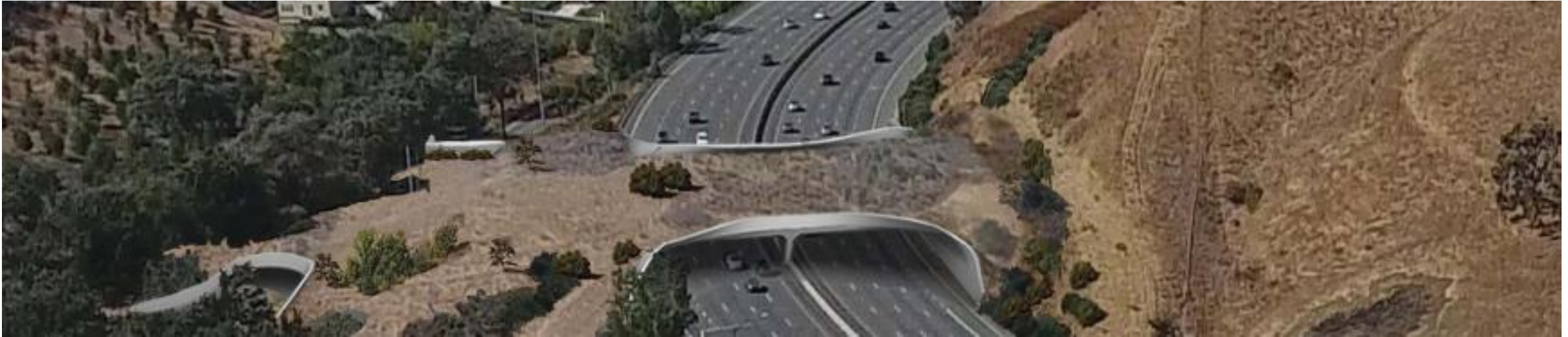
Close up of overpass
