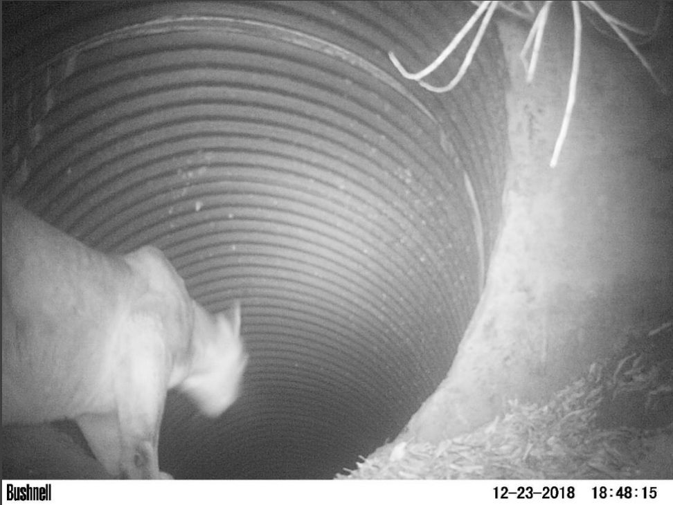
Mountain lion examining culvert under 1-15
