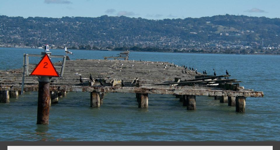
West, distal end of pier where 5000 sq ft of decking will take place, starting behind the timbers and going back about 80 feet, or 5 sets of piling caps.
