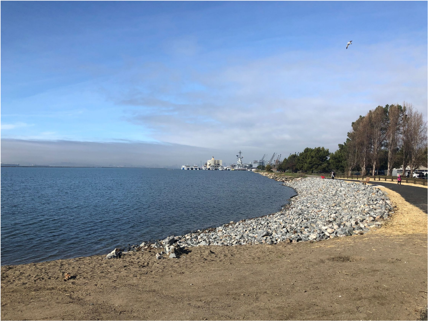
Image 2: AFTER PROJECT: This photo shows the improved shoreline where the derelict barge and concrete debris were once located. The shoreline is now properly stabilized with cobble rip-rap. The public can now safely access the area without the eyesore of shoreline debris (Photo by: East Bay Regional Park District staff).
