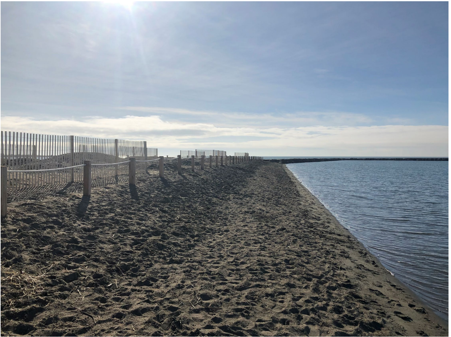
Image 4: AFTER PROJECT: This picture depicts a beach clean of debris. To the left is the dune restoration area. There are two types of fencing seen here: the outside fencing is for site protection and the inner, taller fencing is placed around dune areas to help stabilize the area. Once the dune area is established, the outer fencing will be removed (Photo by: East Bay Regional Park District staff).
