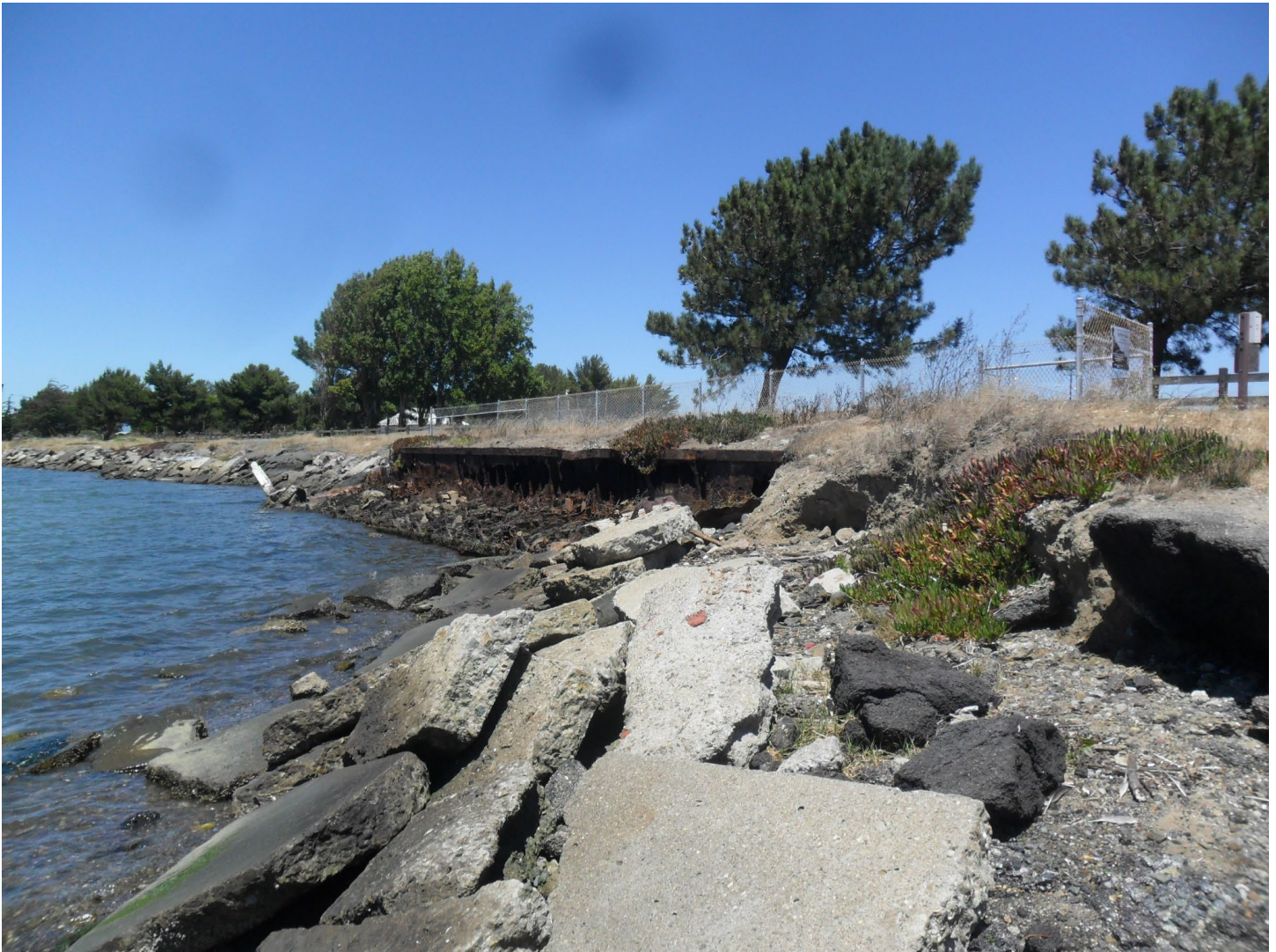
Image 1: BEFORE PROJECT: This picture depicts the derelict barge wedged into the slope of the shoreline. Additionally, concrete debris is also seen here. Both the barge and concrete debris were removed during construction because both were public safety hazards and eyesores. This area of the project is parallel to the Alameda Point Trail (Photo by: East Bay Regional Park District staff).
