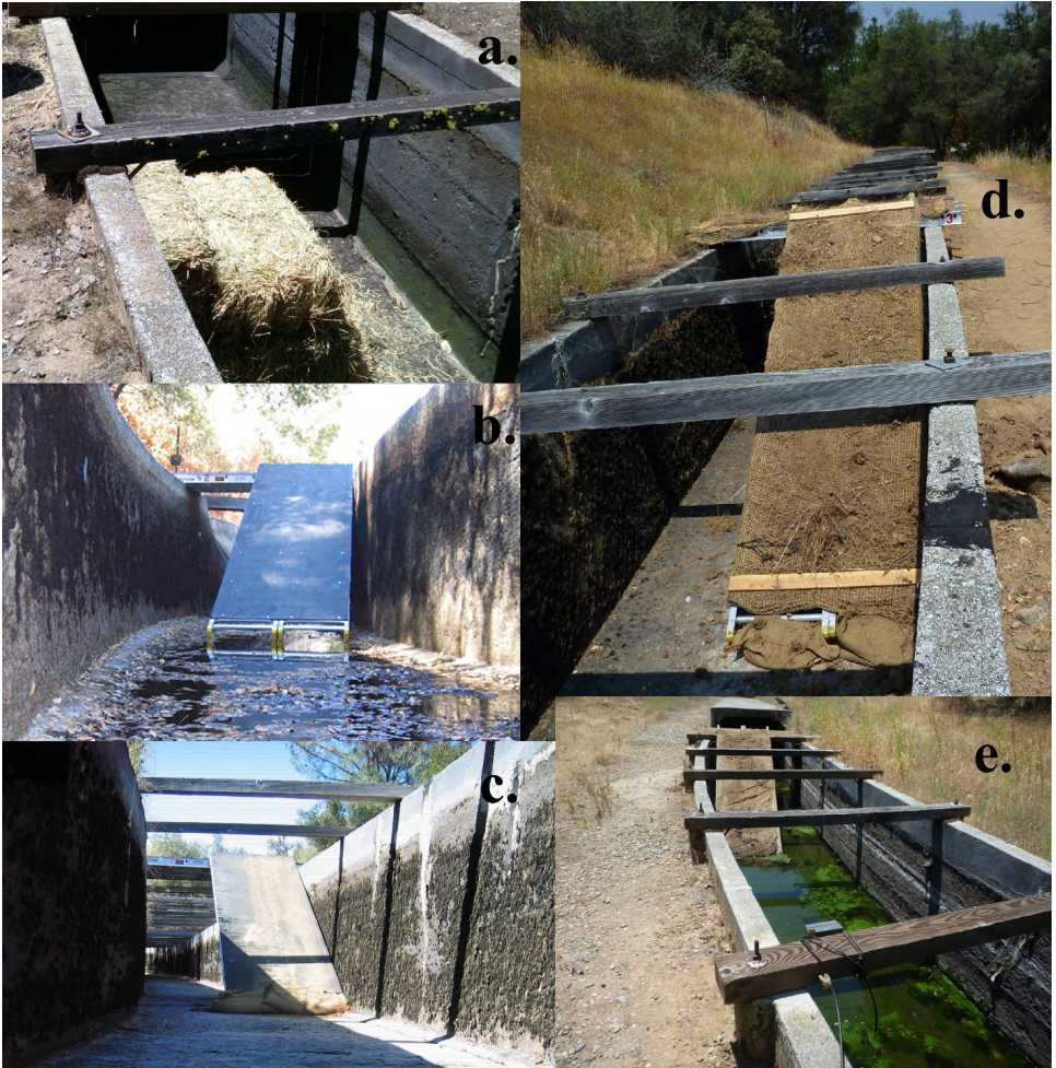
Figure 2. Different iterations of temporary escape structures used from 2011–2018 in canal located in North Fork, California: (a) Hay bales arranged in step configuration (2011), (b) Aluminum platforms covered with rubber sheets (2012), (c) Aluminum platforms covered with rubber sheets and sandbags installed at base of ramp (2012), (d) Aluminum platforms covered with rubber sheets, sandbags deployed at base of ramp, and jute netting and debris utilized (2013), (e) Aluminum platforms covered with rubber sheets, sandbags deployed at base of ramp, jute netting and debris utilized, and camera trap attached to canal crossbeam (2017).
