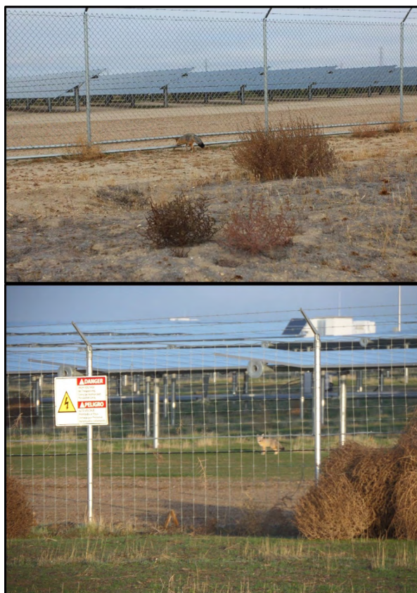
Figure 2. Images of security fences that are permeable to San Joaquin kit foxes at the Topaz Solar Farms (a kit fox is visible crossing through the gap at the bottom of the fence) and California Valley Solar Ranch (a kit fox that just crossed through the fence is visible inside the facility) in San Luis Obispo County, California. (Top photo by Larry Saslaw; bottom photo by Christine Van Horn Job.)
