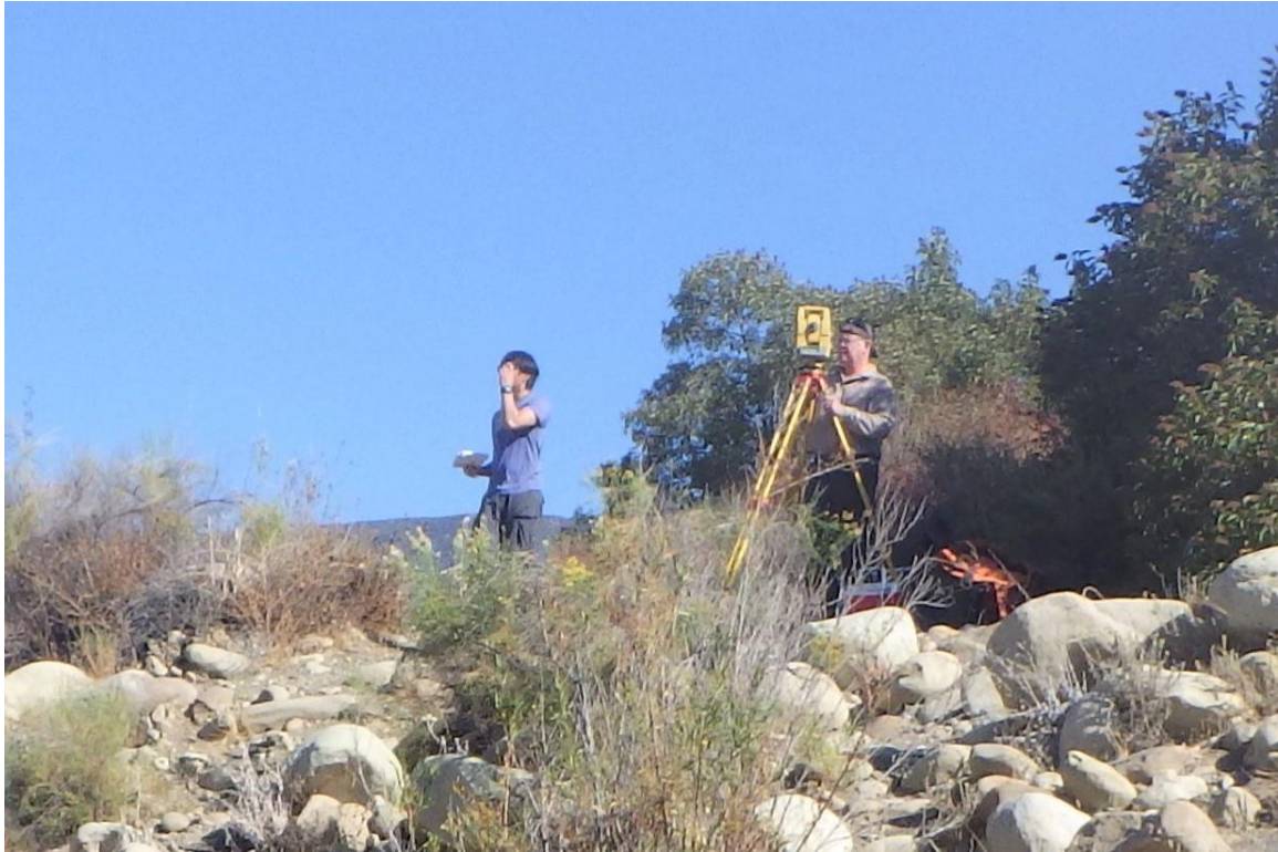
Figure 13. Collecting terrain model data in the study site using a total station.
