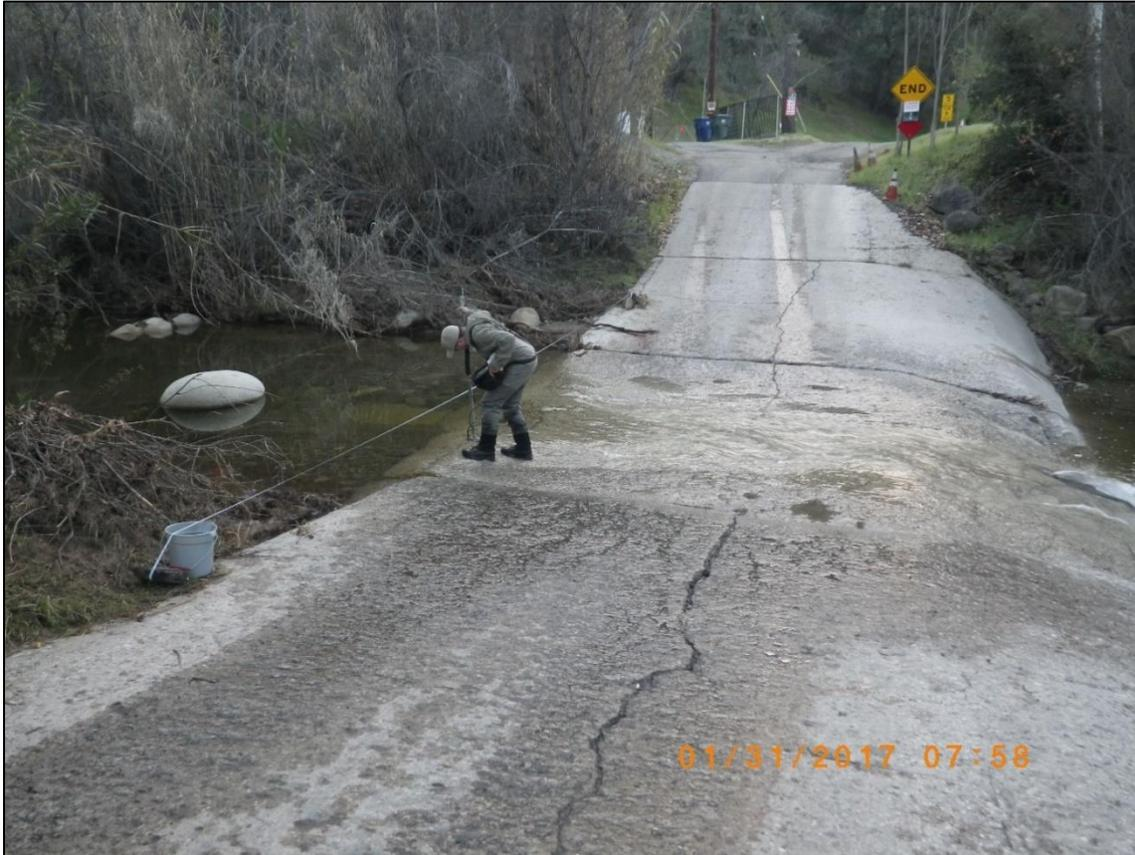
**Figure 6.** Photo of a partial passage barrier at the Fraser Street Arizona crossing. Flow pictured at approximately 2 cfs.
