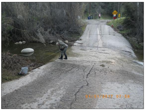
**Figure 6.** Photo of a partial passage barrier at the Fraser Street Arizona crossing. Flow pictured at approximately 2 cfs.
