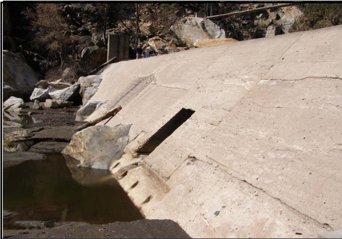
Figure 5. Escondido Canal diversion dam (RM 40).
