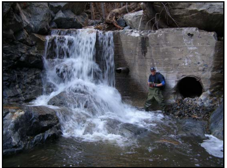
Figure 8. Steelhead/trout barriers on lower Pauma Creek.
