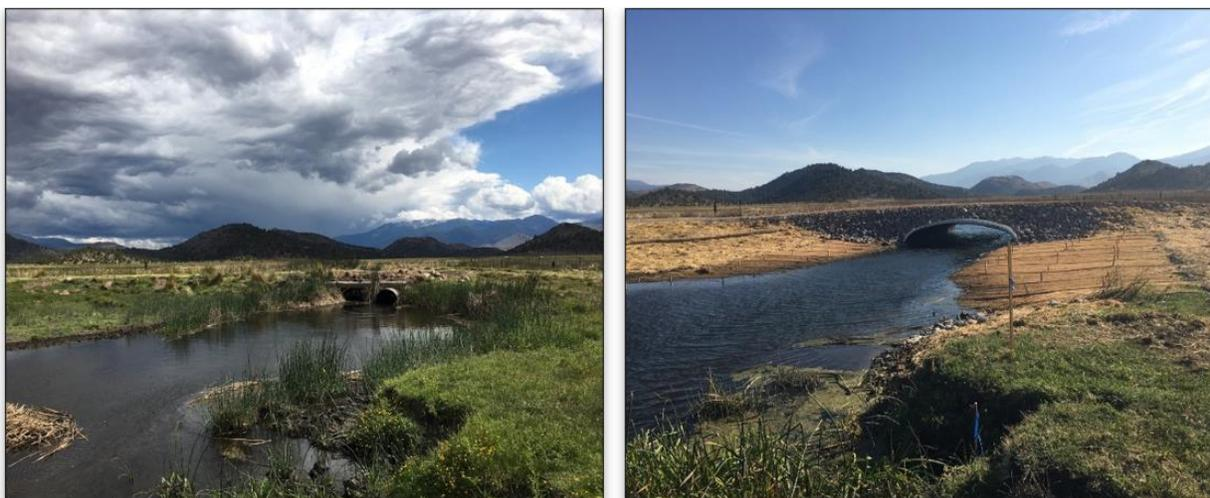
*Figure 3. The Parks Creek culvert before (left) and after (right) restoration work, viewed from downstream (credit: AquaTerra Consulting LLC)*
