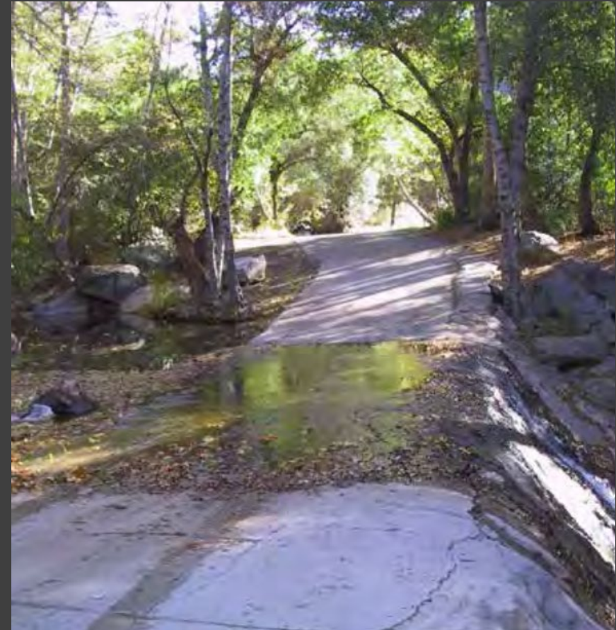
Crossing to be replaced by clear span bridge
