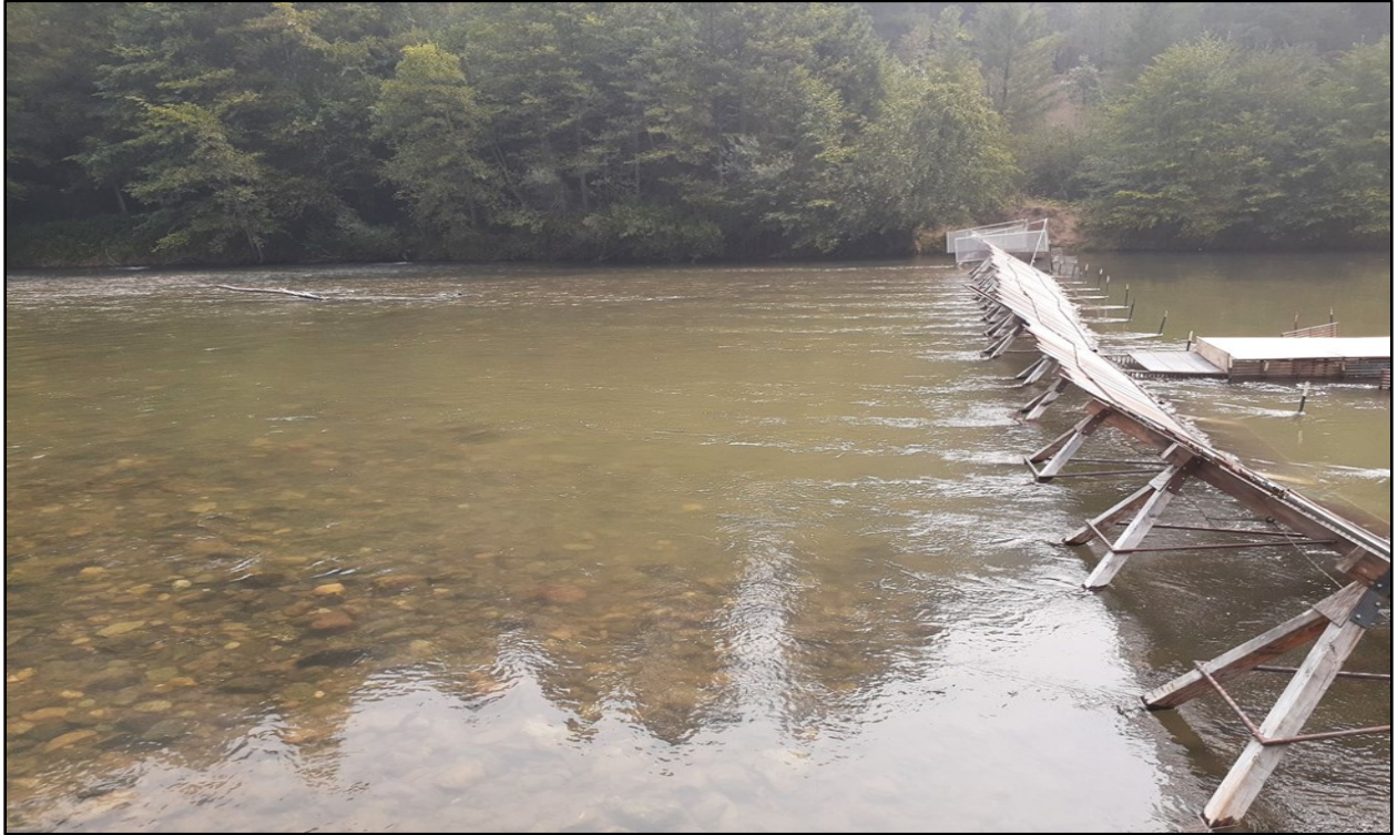
Figure 3. Junction City weir configuration in 2020. This shows the weir in trapping mode. Flow is right to left. The water turbidity is a result of upstream restoration work.
