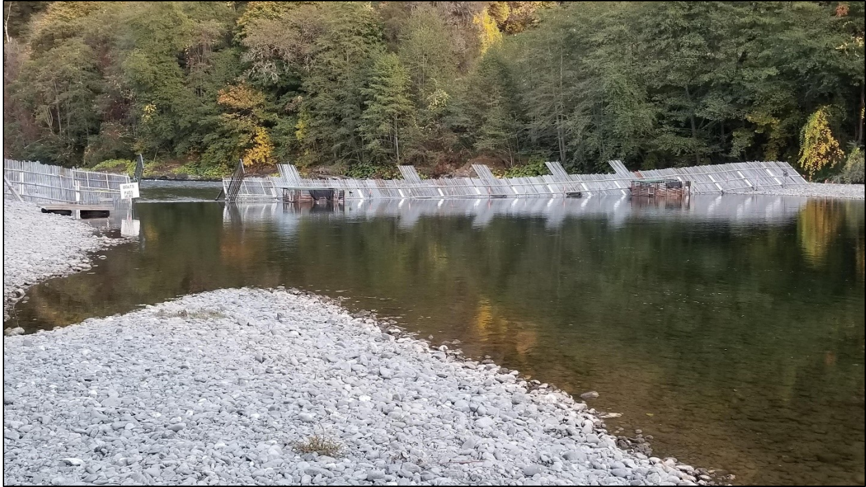
Figure 4. Willow Creek weir in 2020 (in “open” mode), with standard boat gate and two traps. Flow is from right to left.
