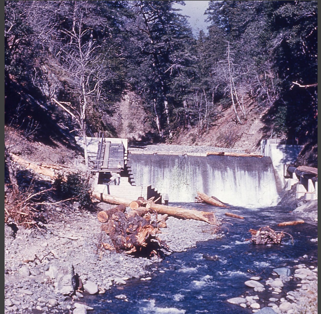
Cedar Creek Dam and Ladder at Hatchery Circa 1960
