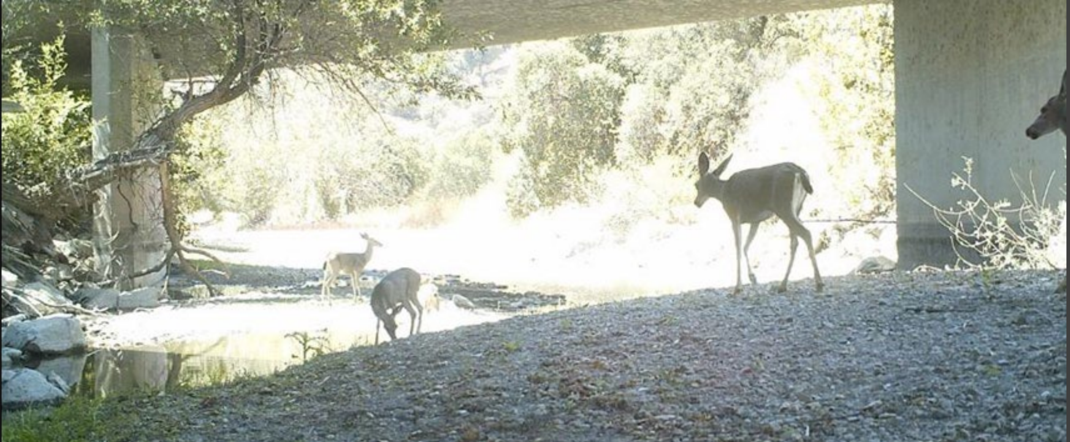
Deer using passage under the midsection of the SR-152 Pacheco Creek Reserve Bridge
