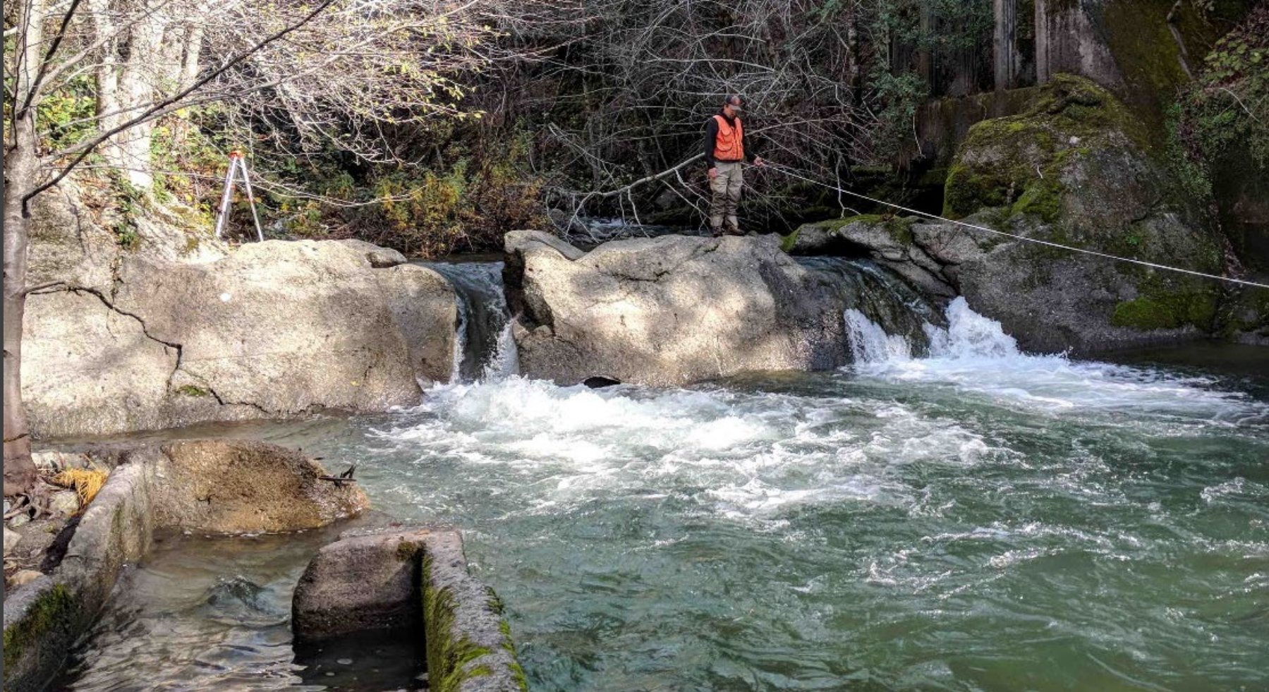
Concrete Diversion Dam
