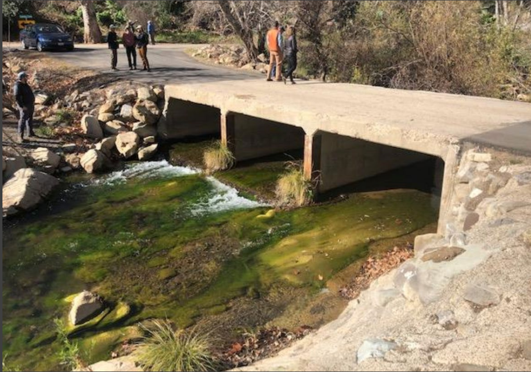
Camino Cielo Bridge
