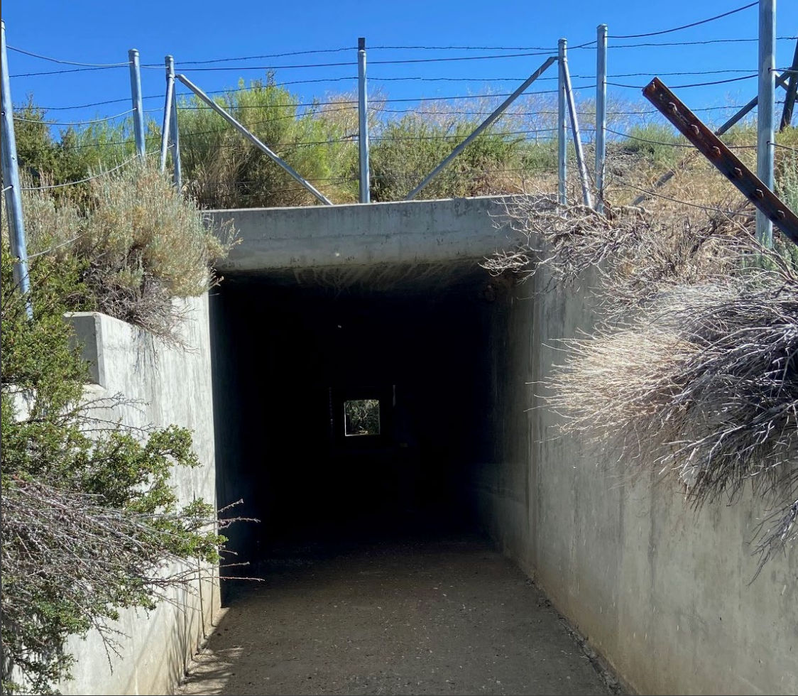
Culvert Under U. S. Highway 395
